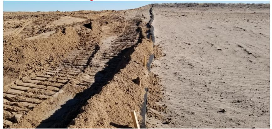
**Photo 4.** Photo taken from the southern perimeter of the location, facing East. Photo depicts soil pushed over the filter fabric BMP .
