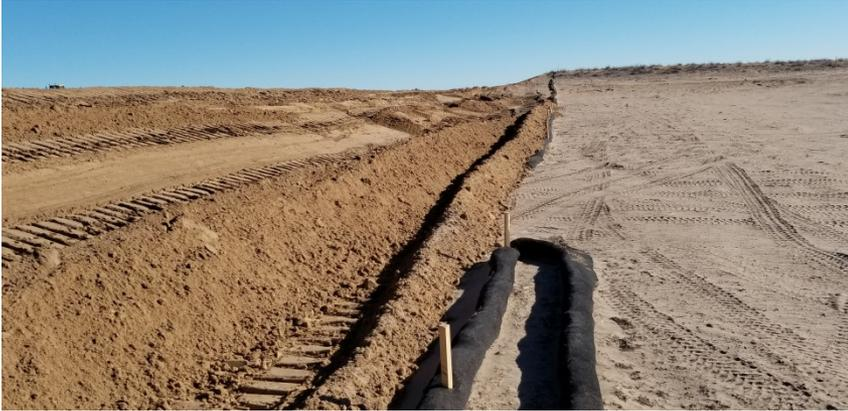
**Photo 3.** Photo taken from the southern perimeter of the location, facing East. Photo depicts breaks in the perimeter of the filter fabric BMP .
