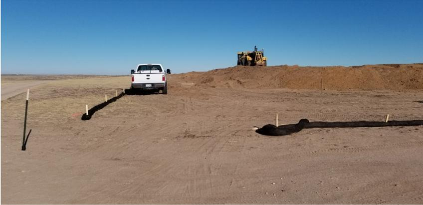
**Photo 1.** Photo taken from the southwestern perimeter of the location, facing North. Photo illustrates a Filtrexx BMP that has been installed around the perimeter of the location.
