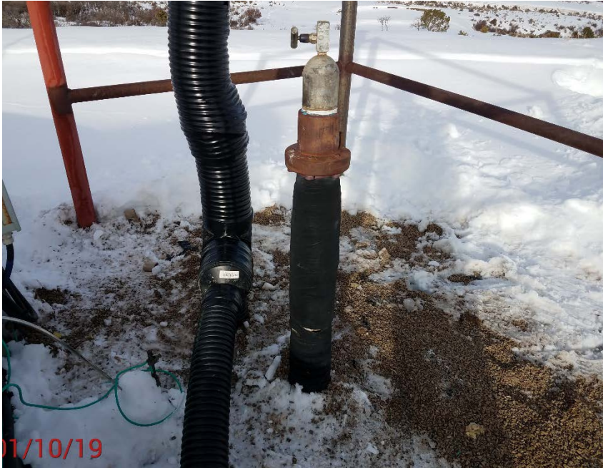
Location Photo #3, Unused Flow line riser on North end of battery.
