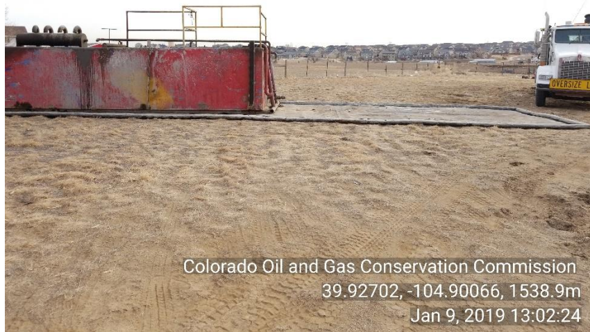
Photo 9 Cleaned up fluid and installed liner under tank
