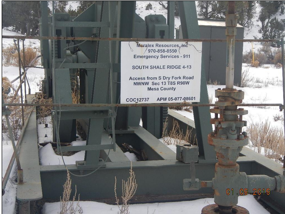
Well head signs in place
