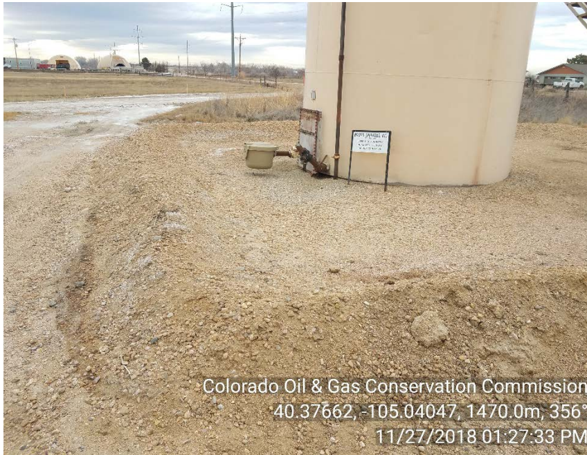
Crude oil tank berm on 11/27/18
