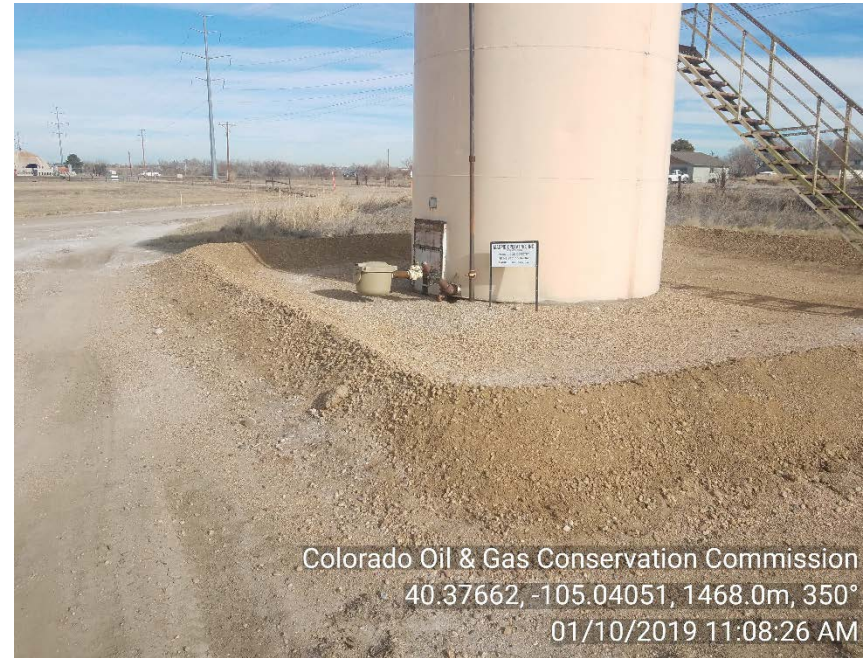
Crude oil tank berm on 1/10/19
