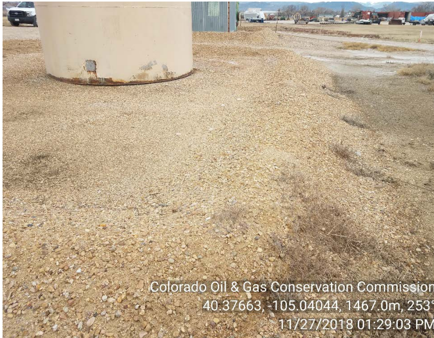
Crude oil tank berm on 11/27/18
