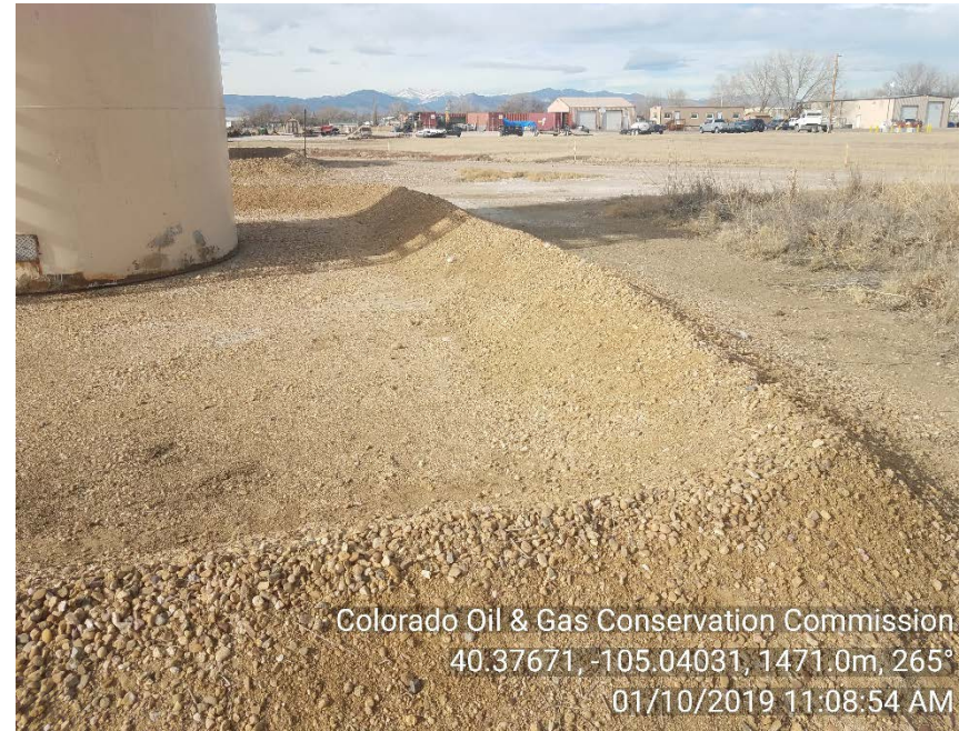
Crude oil tank berm on 1/10/19
