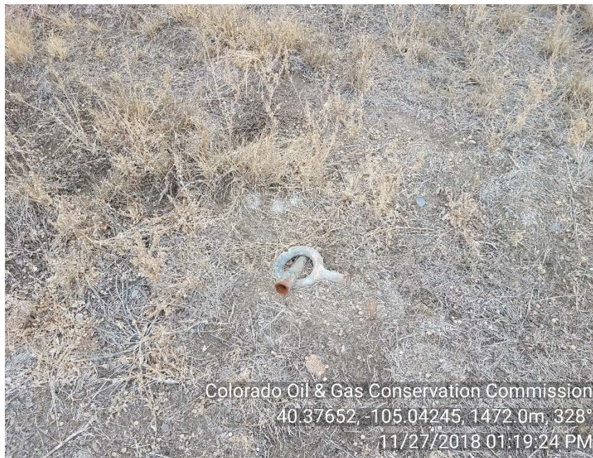
NW deadman on 11/27/18
