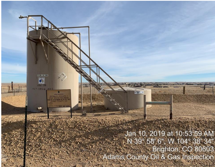
Photo#1 Production Tank and Produced Water Pit
