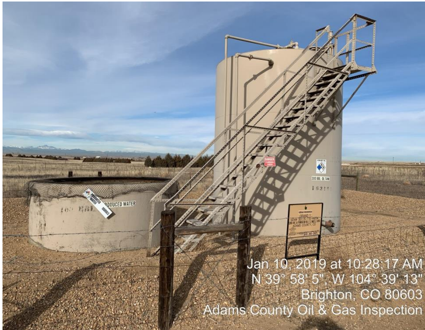
Photo#1 Production Tank and Produced Water Pit
