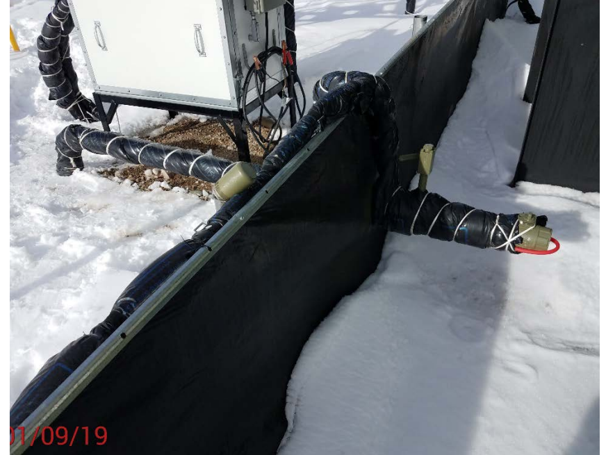
Location Photo #2, Unused flow line on west end of tank battery.
