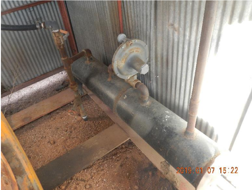
Photo 13: Horizontal supply gas knock out with black poly supply gas line coming in from top L and 1" steel line out bottom to unknown point.
