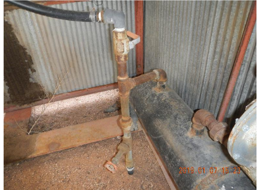
Photo 14: Close up of supply gas knock out.
