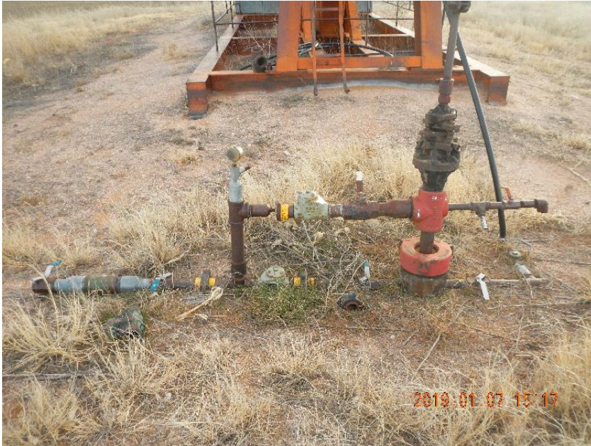
Photo 5: Wellhead tree.
