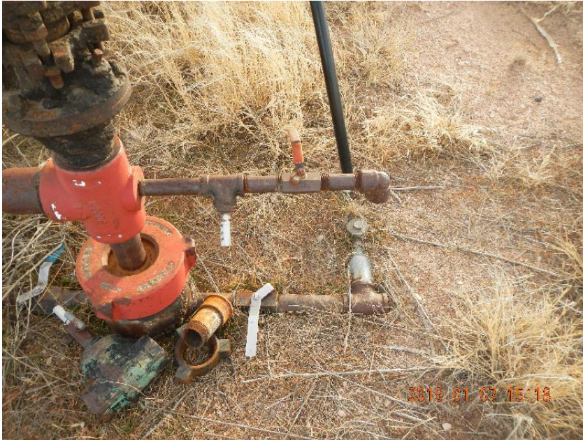
Photo 7: Above ground supply gas line off wellhead casing.
