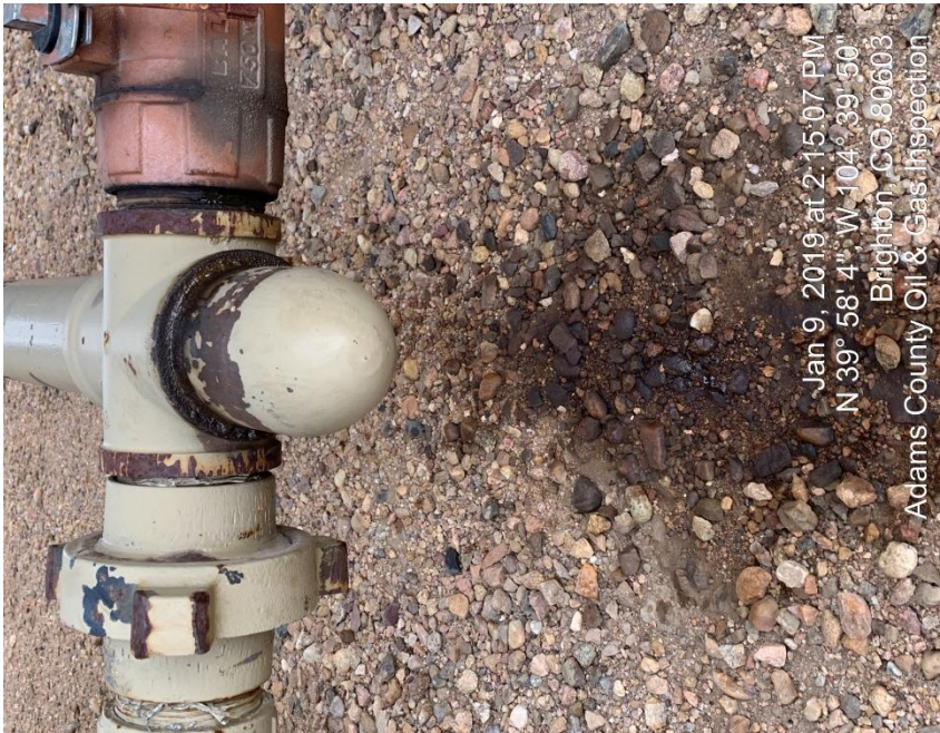
Photo#7 Corrective Action/Leak
