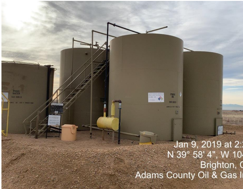
Photo#1 Production Tanks/Produced Water Tank
