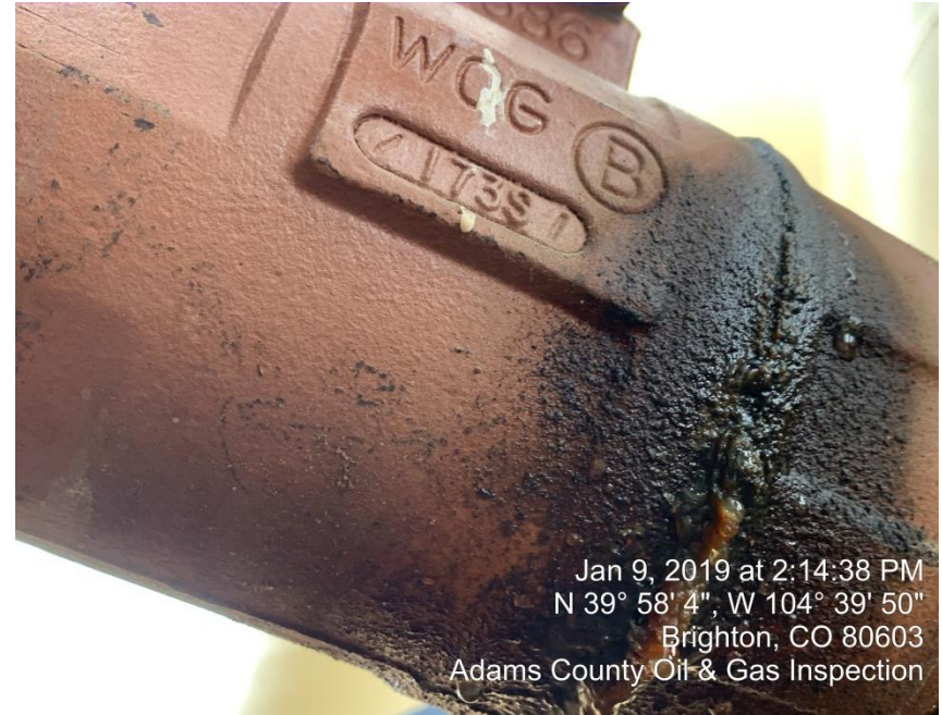
Photo#6 Corrective Action/Leak
