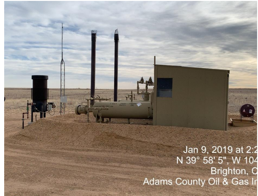
Photo#2 (2)Separators/ECD/2 Gas Meters/Automation RTU
