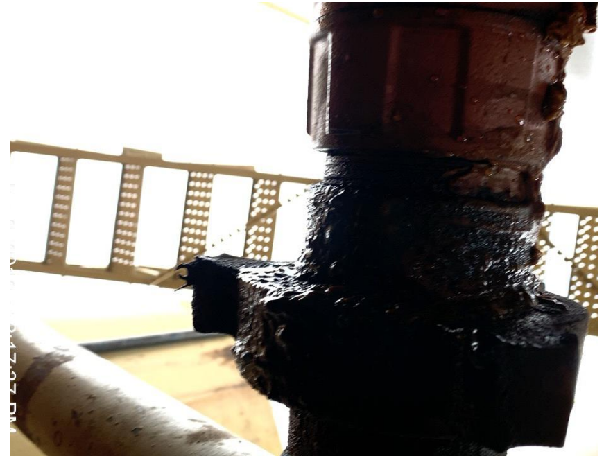
Photo#10 Corrective Action/Leak
