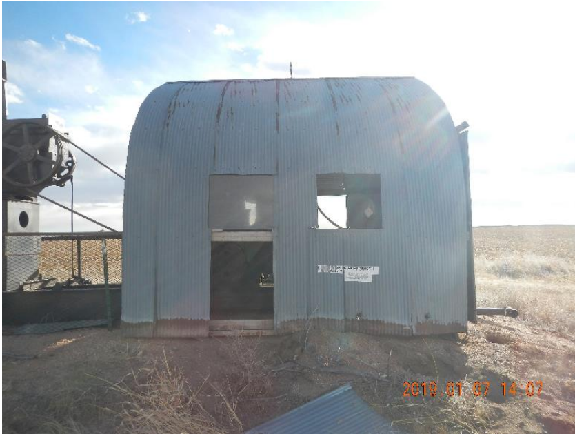
Photo 9: Steel building over prime mover.
