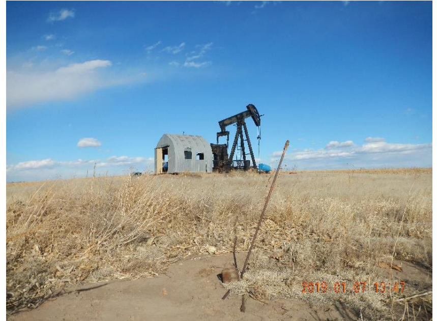
Photo 2: One of (4) anchors with pump jack in back ground.
