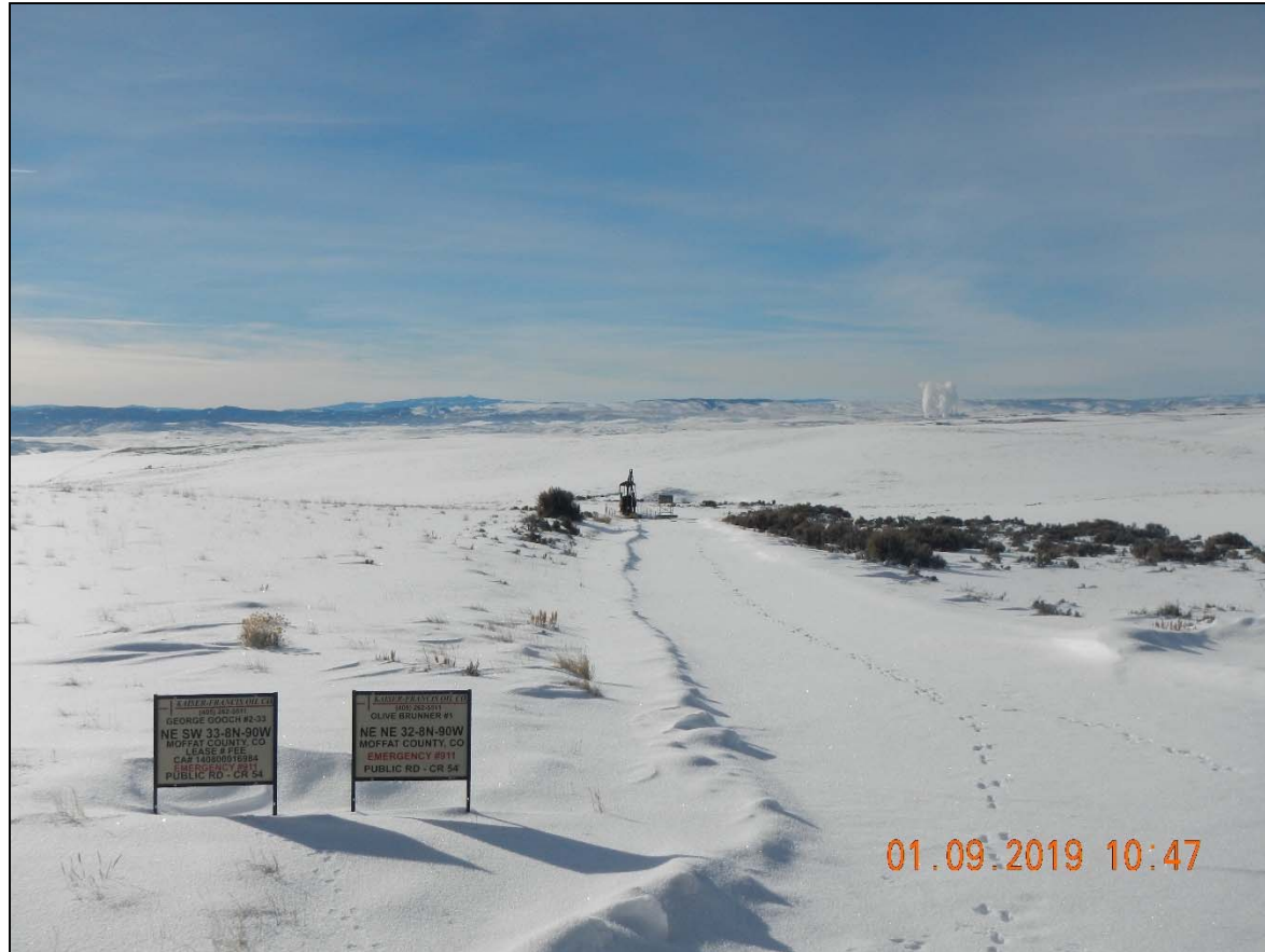
Photo 1. Overview of road where maintenance stops.
