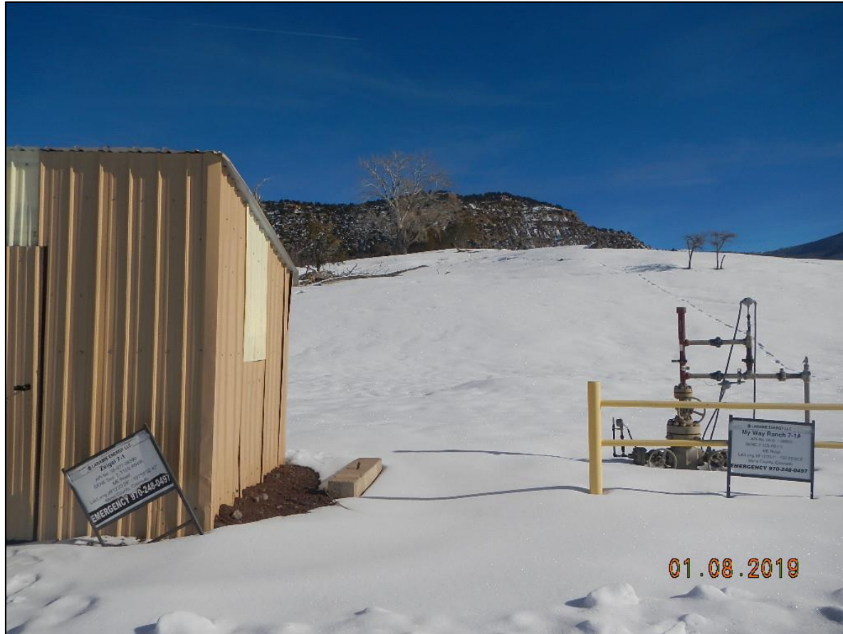
Well head signs in place
