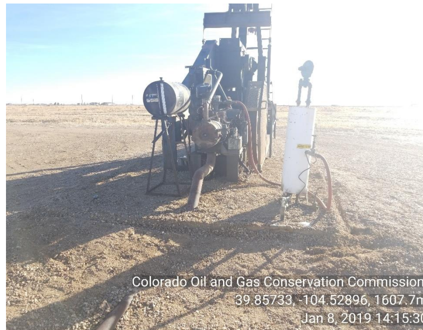
Photo 2 Stained soil removed
