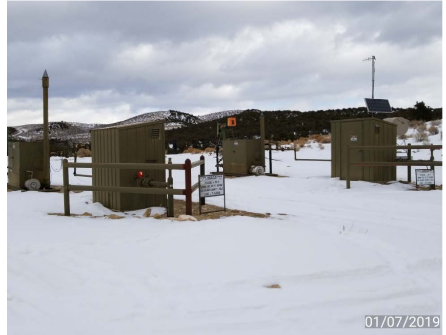
Photo 2. Separators and gas meter buildings.
