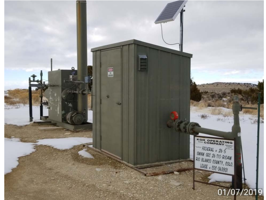
Photo 2. Gas meter building and separator.
