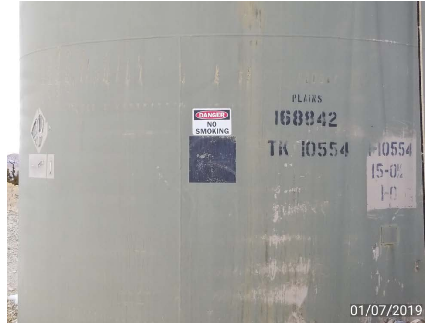
Photo 4. Tank NFPA / contents / capacity label missing.
