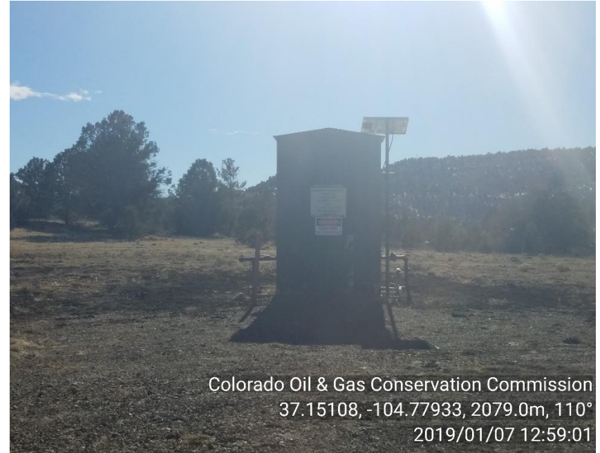
PHOTO 2: WELL SIGN/METER HOUSE
