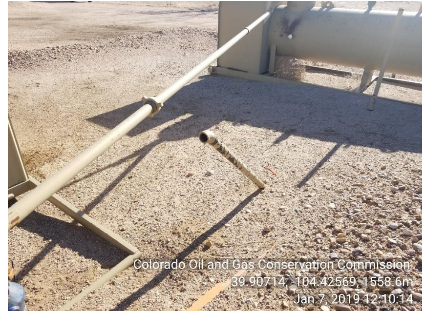
Photo 8 unmarked riser between sep and meter house
