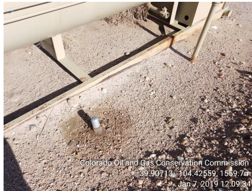
Photo 4 Stained soil 2" line next to separator
