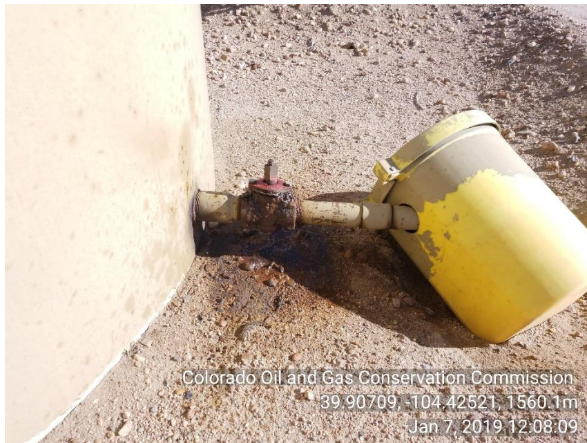
Photo 3 leaking VLV and stained soil crude oil tank #75110
