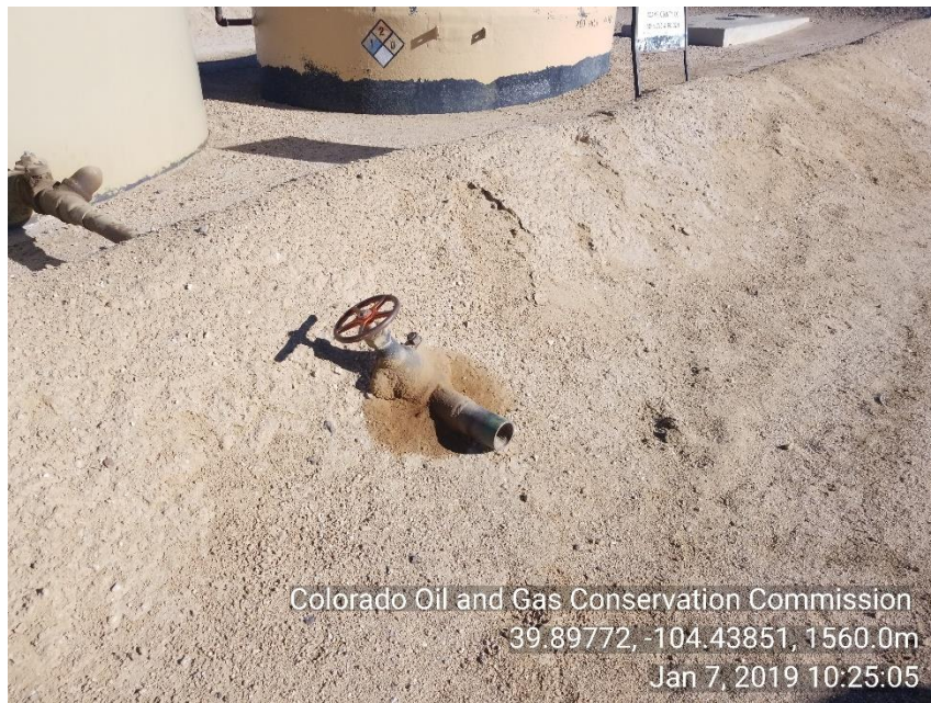
Photo 5 Stained soil around load VLV
