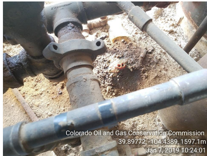
Photo 6 Stained soil in seperator
