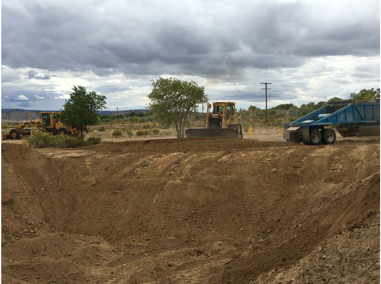
Photo 9: Clean import soils were delivered for backfill activities.
