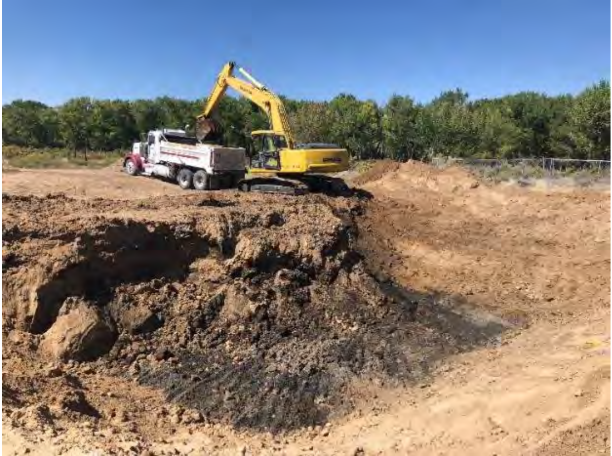
Photo 4: Excavator direct loads dump truck with impacted soils.
