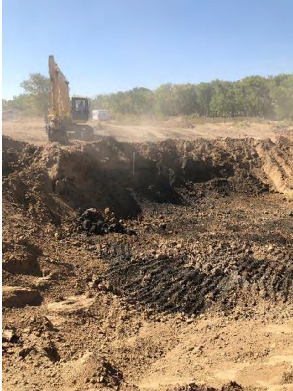
Photo 5: Removal of impacted soils near decommissioned MW-01.
