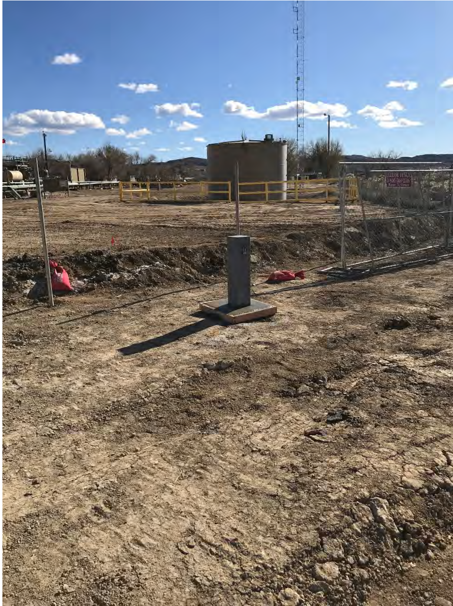
Photo 11: MW-01R installed.
