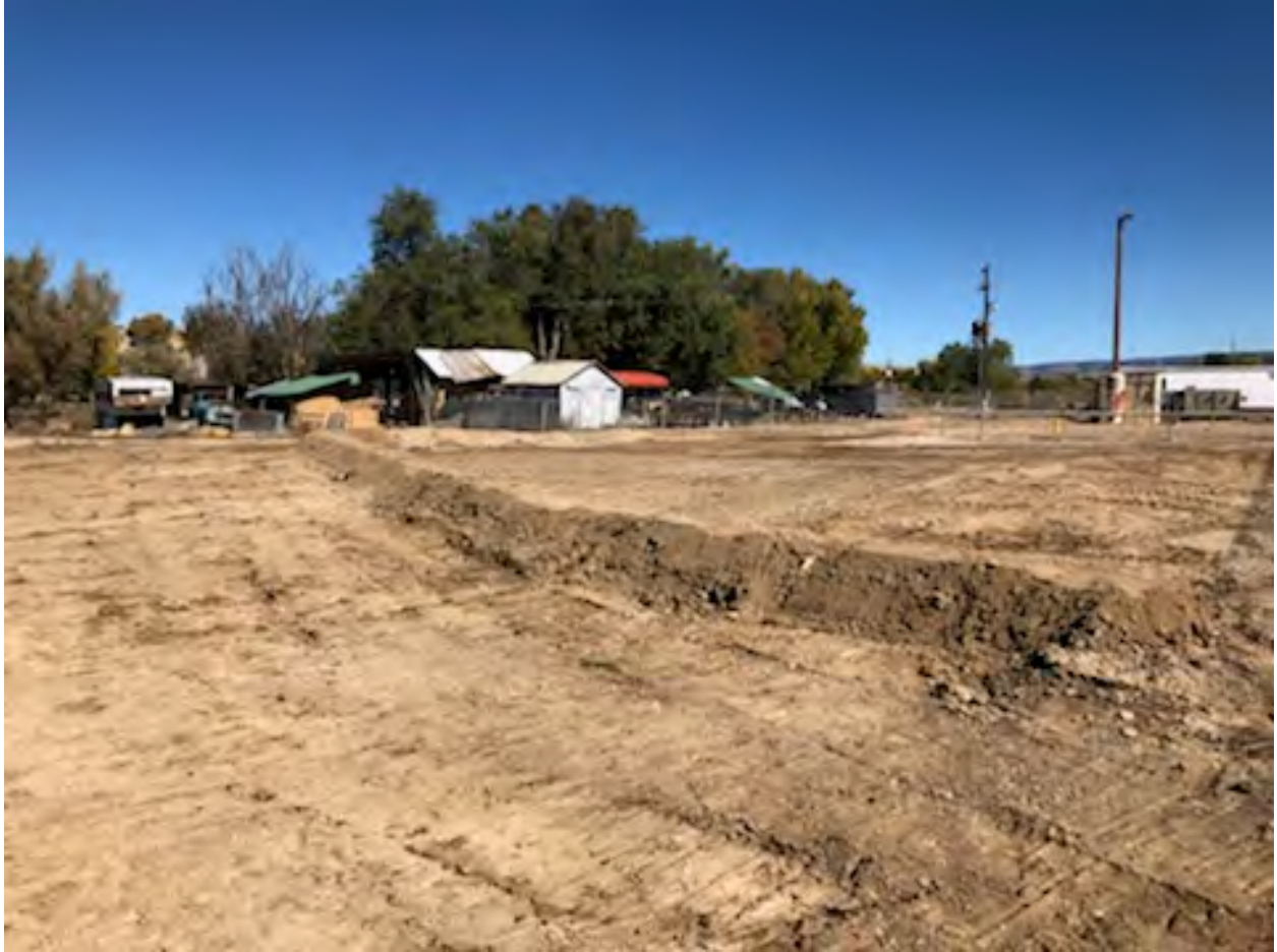
Photo 10: Site restored and stormwater berm in-place.
