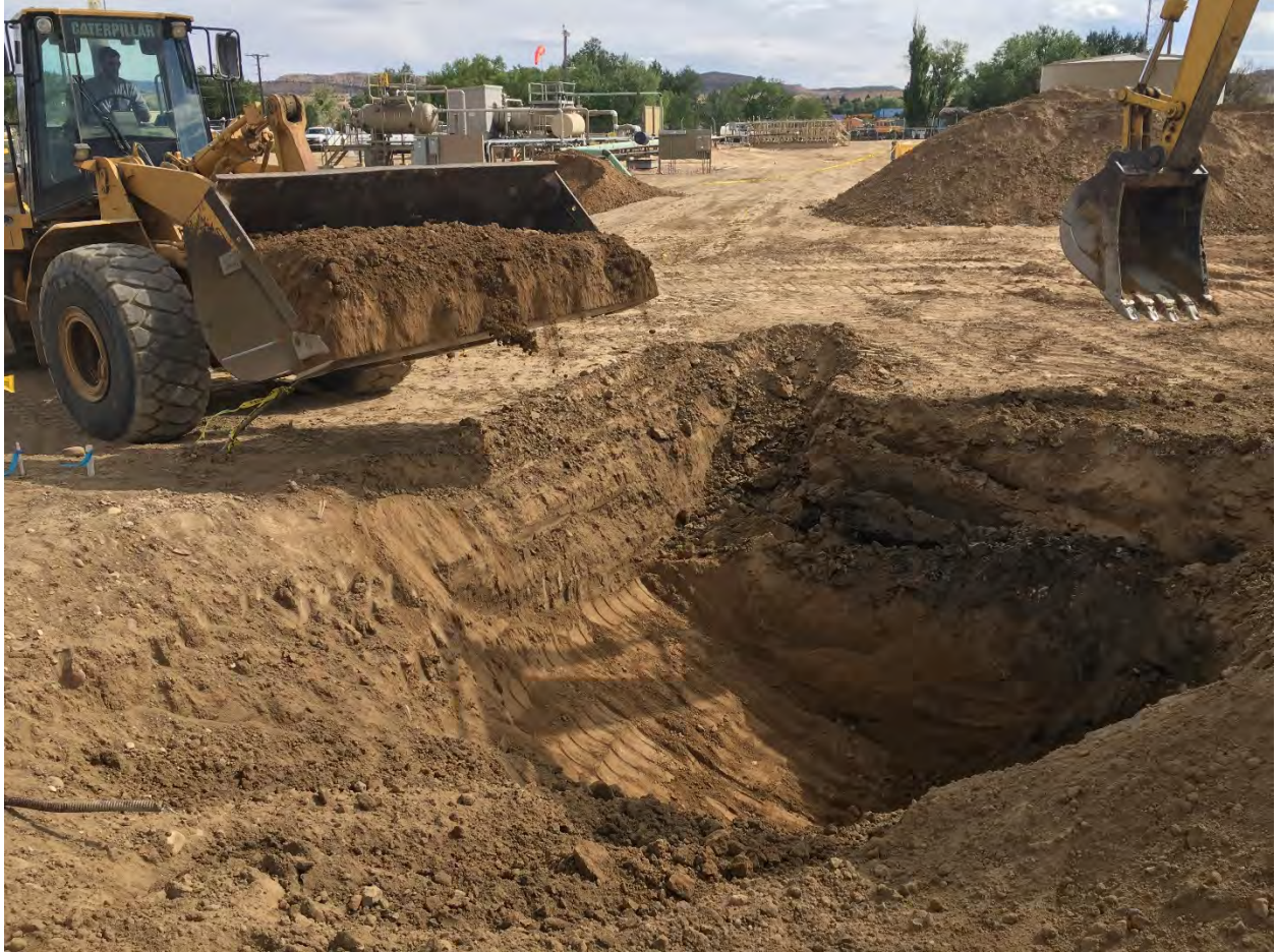
Photo 3: Clean backfill was placed in the excavation trench, following removal of impacted soils, to protect active utilities.
