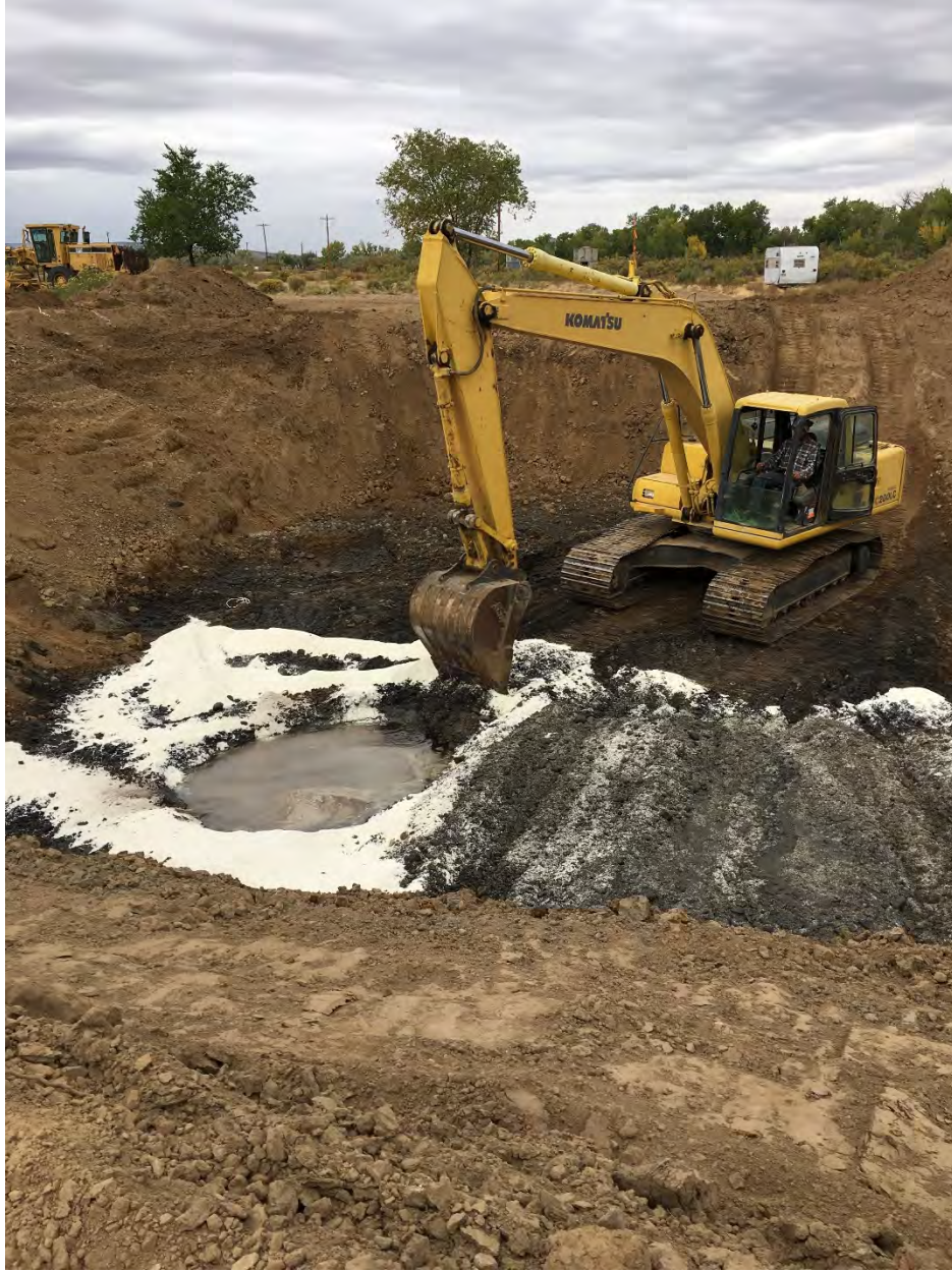
Photo 8: Calcium nitrate was spread across the bottom of the excavation floor and mixed into the gravel layer.
