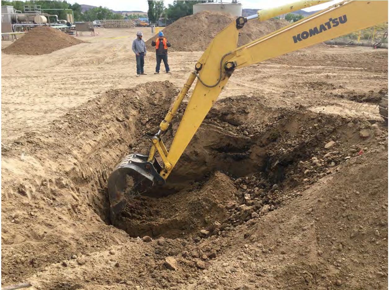
Photo 2: Rolling excavation trench methods were used along the eastern edge of the excavation to protect active utilities.
