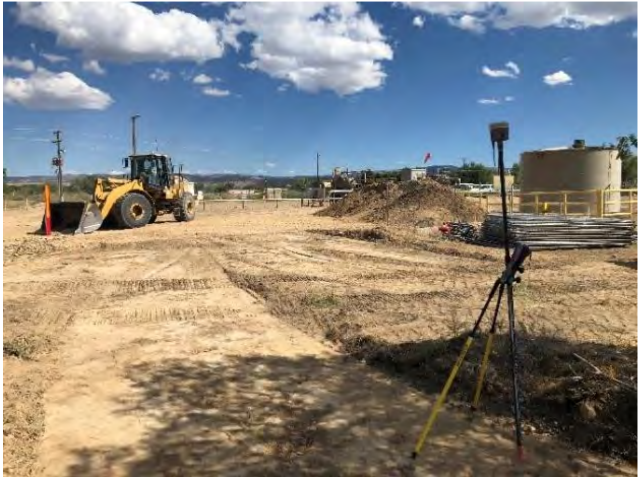
Photo 1: Using survey control to stakeout limits of clean overburden material. Loader strips and stockpiles clean material on-site.
