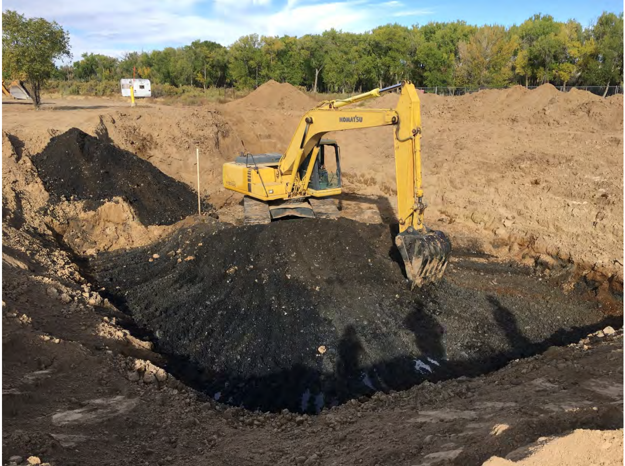
Photo 6: An additional 1-foot of gravel material was removed from the excavation floor to reach the top of the groundwater table.
