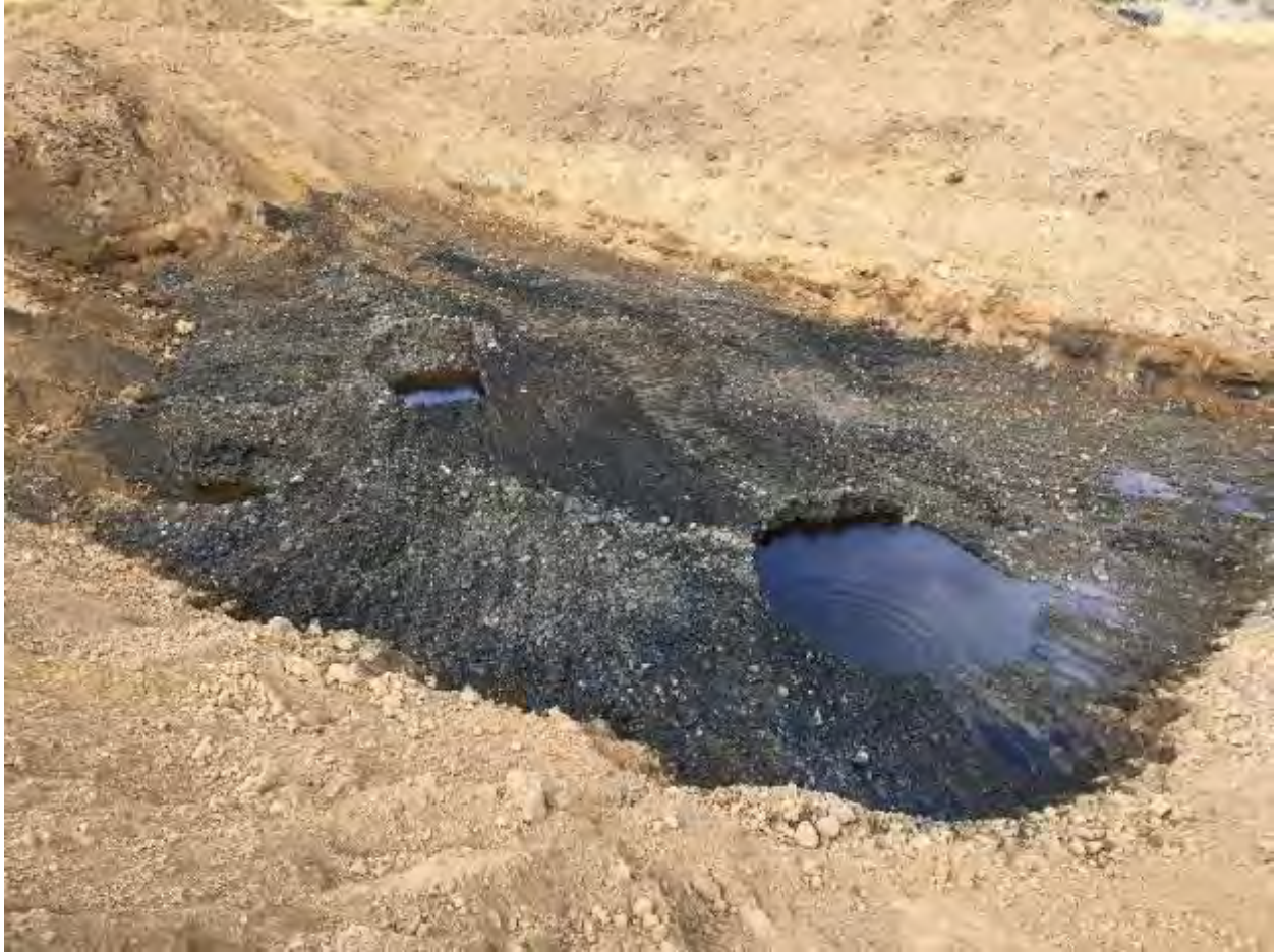
Photo 7: Three sumps were excavated into the excavation floor and liquids were removed with a vacuum truck.
