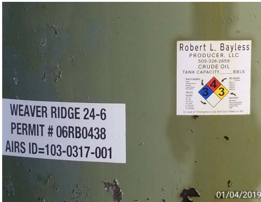
Photo 5. Tank missing capacity volume of 300 bbl.
