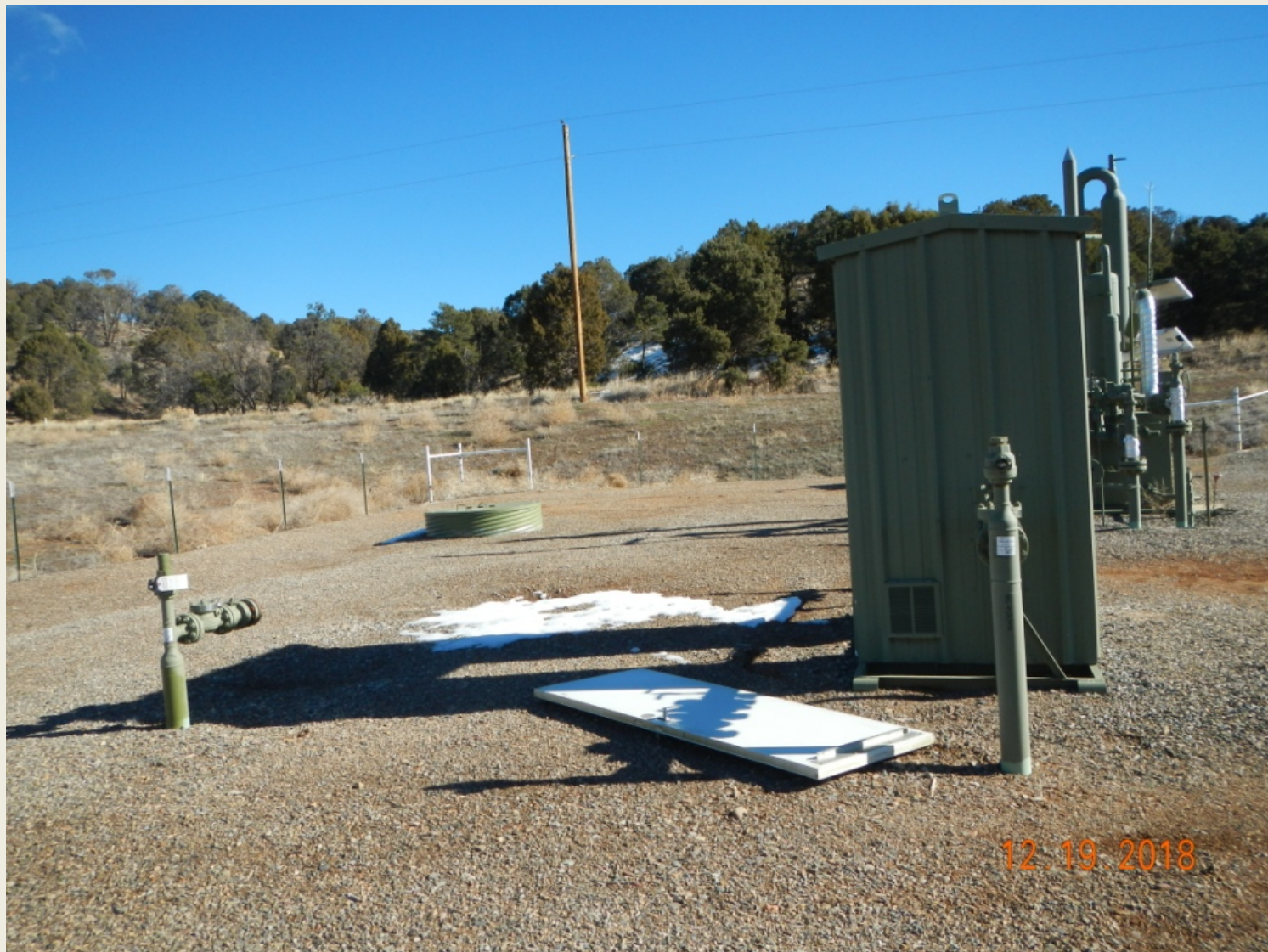
Photo 2. View of more risers on active location. Not apparent whether all risers are associated with producing well or whether some are remaining from PA well.
