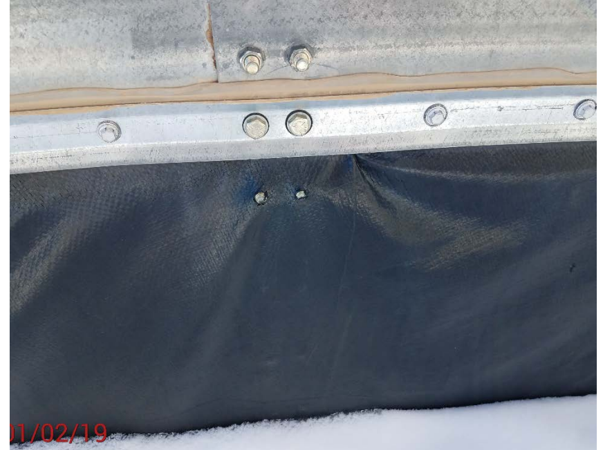
Location Photo #4, Holes in secondary containment liner.
