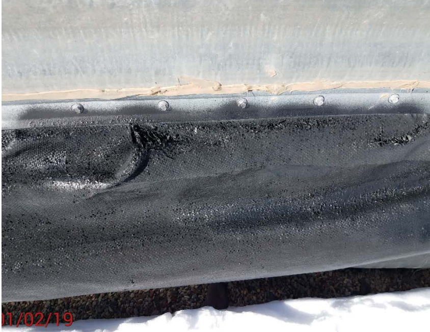
Location Photo #3, Holes in secondary containment liner.
