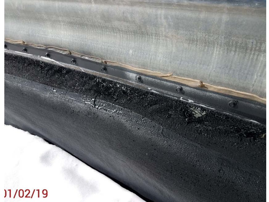
Location Photo #2, Holes in secondary containment liner.
