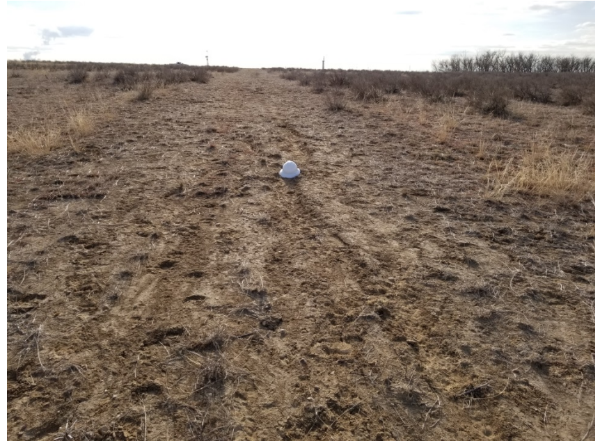
Photo 4. Photo taken from the access road, facing Southwest. Photo depicts apparent start of rill erosion along access road.
