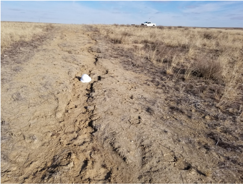
Photo 5. Photo taken from the access road, facing Northeast. Photo depicts apparent rill erosion along access road.
