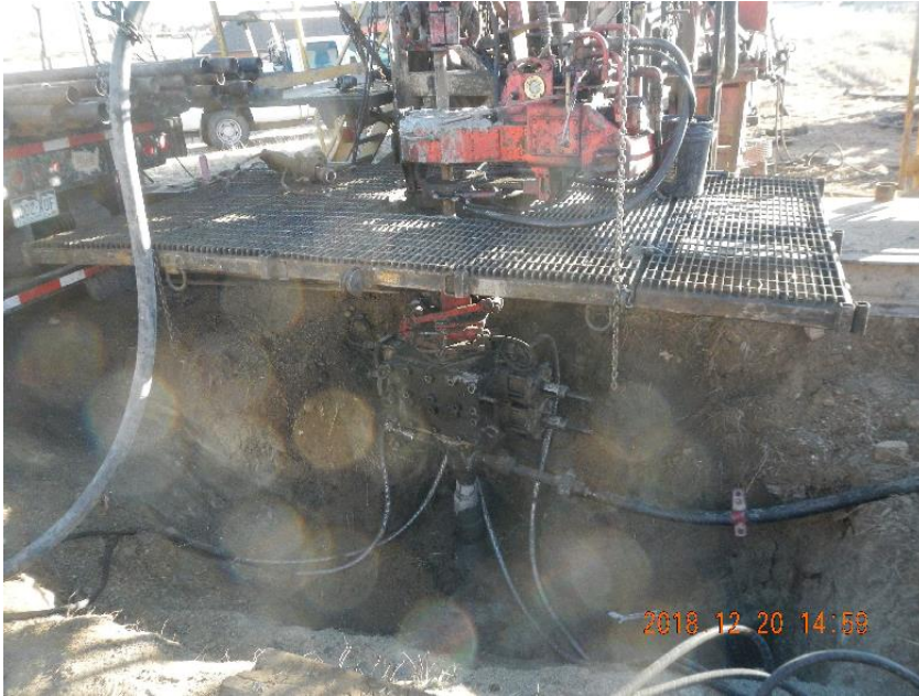
Photo 3: Rigged up to casing for returns while pumping cement.
