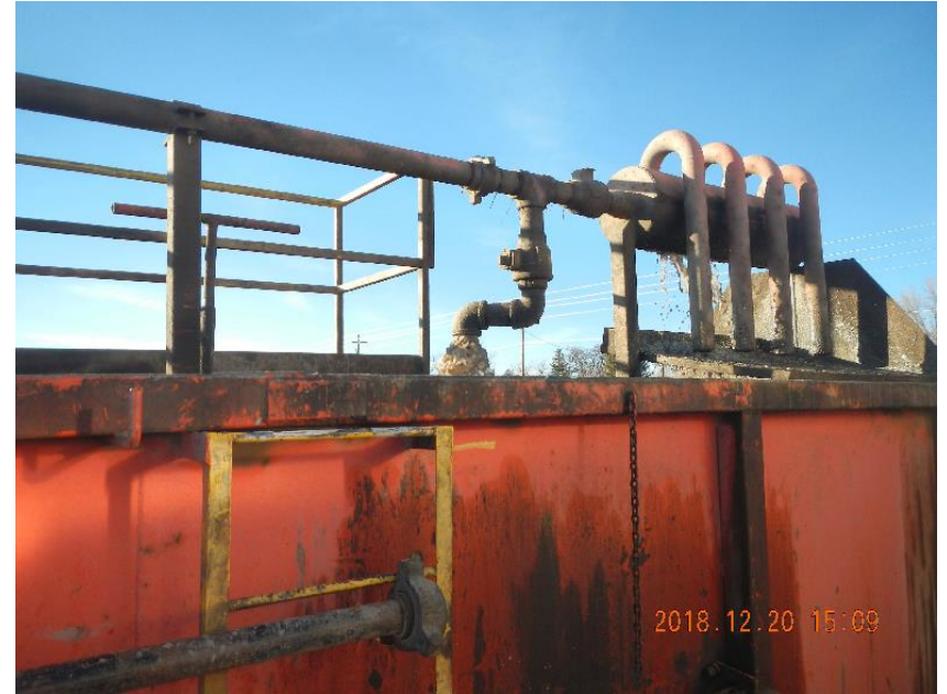
Photo 4: Returns to tank during cementing operation.
