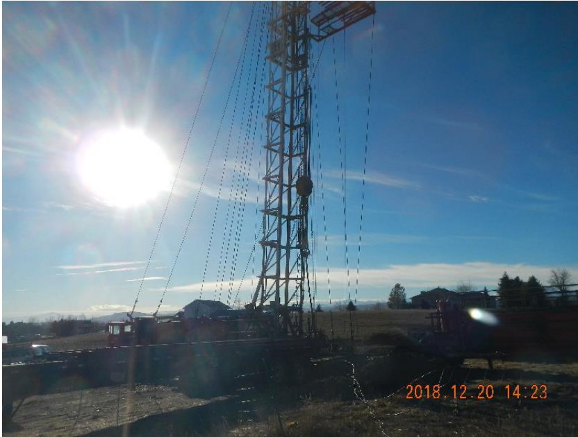
Photo 1: Rig 9 on well for P&A operation.
