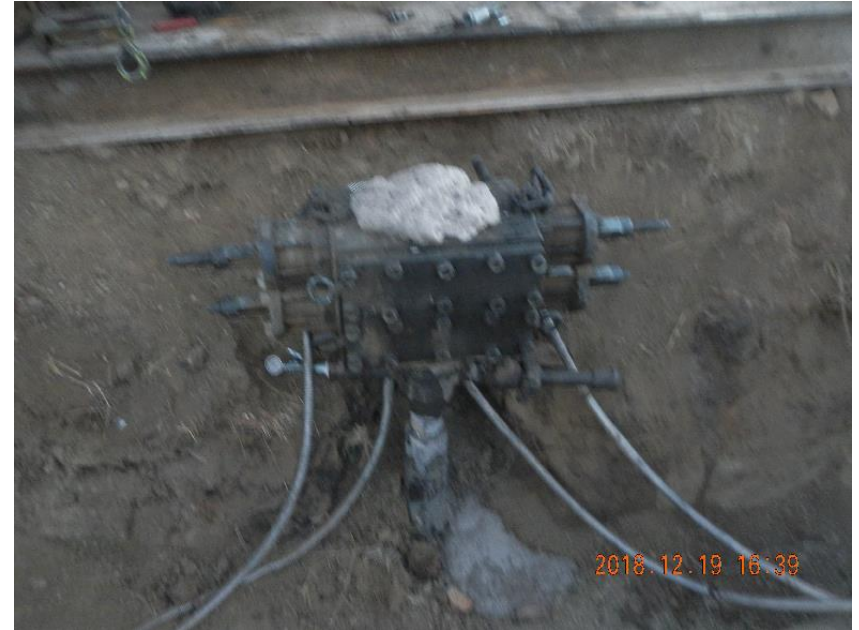
Photo 8: BOP installed and well control established.
