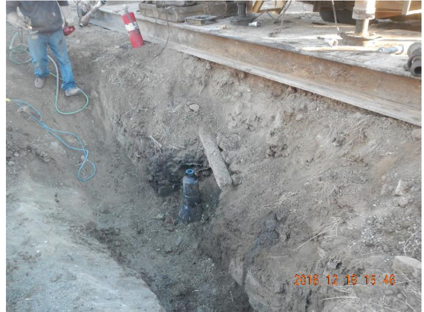
Photo 6: Well dead and 2" pipe portion of the wellhead cut off.
