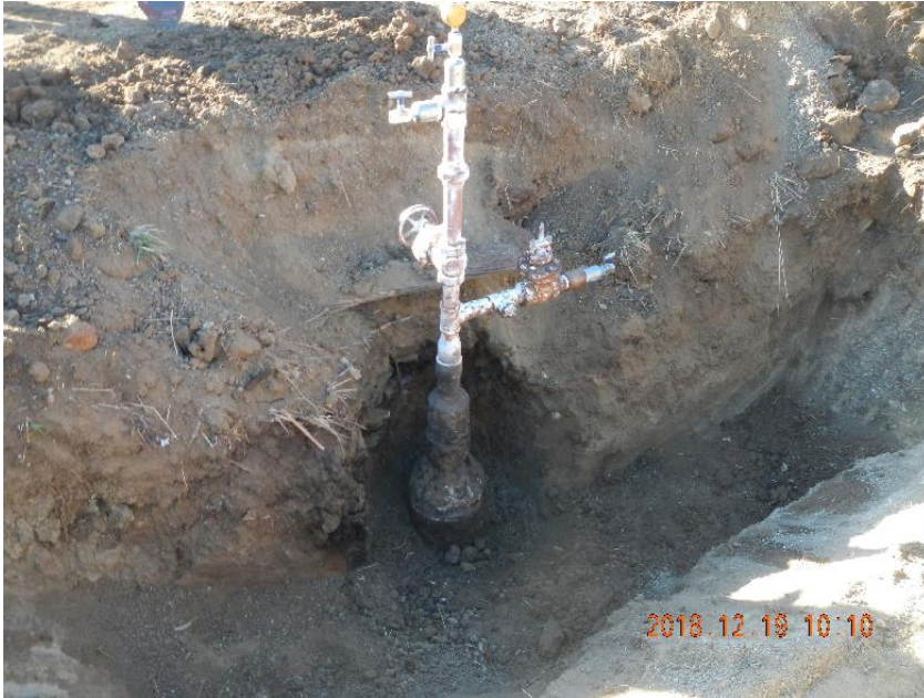
Photo 1: Excavation trench on N side of wellhead.
