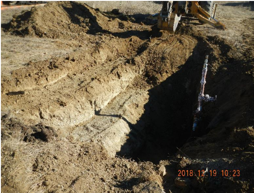
Photo 3: Overview of excavation on N side of wellhead.
