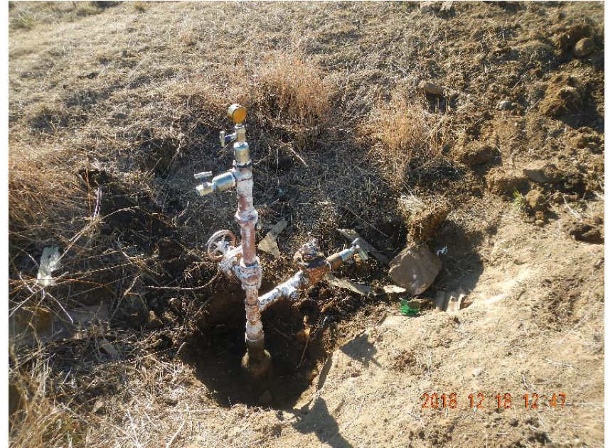
Photo 8: Beginning of excavation around base of wellhead looking for surface casing.
