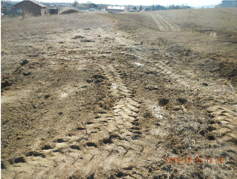
Photo 7: Backfilled area on W side of wellhead.
