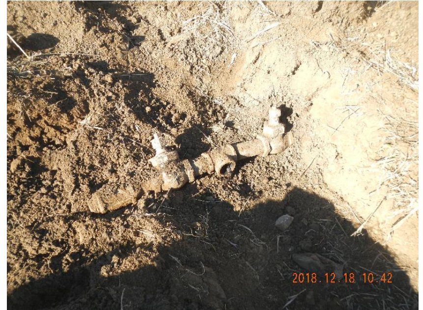
Photo 2: W 2" flowline T running N and S.
