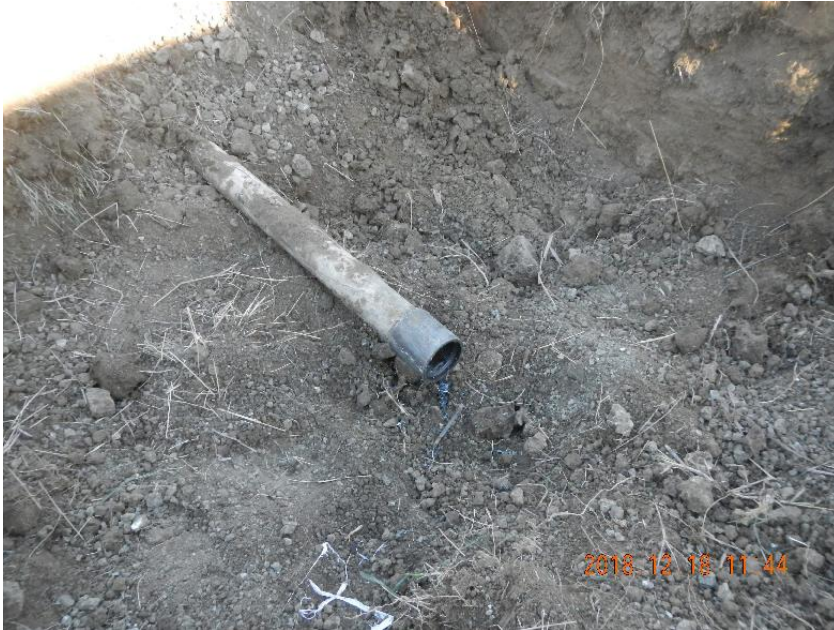
Photo 3: 2" flowline cut and threaded with collar installed.
