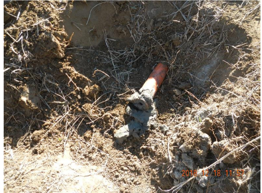
Photo 6: 1" orange poly line sealed with foam plug, cement, and foam plug for landowner.
