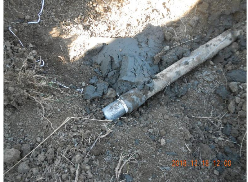
Photo 4: 2" cemented flowline abandonment completed with bull plug installed.
