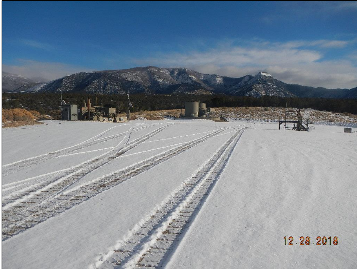
Photo from N side of location
