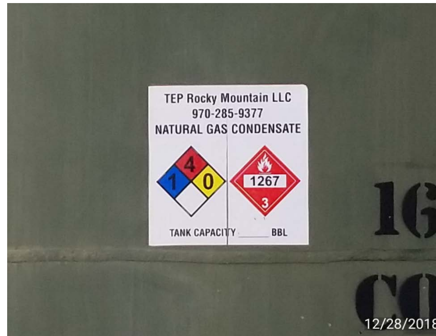
Photo 2. Tank label volume capacity is illegible.
