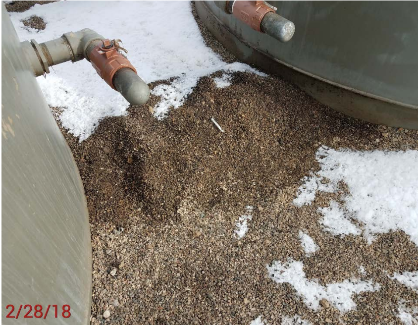
Location Photo #3, Stained rock in battery containment.
