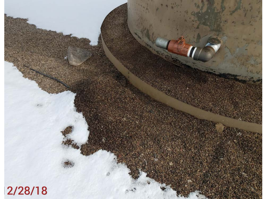
Location Photo #2, Stained rock in battery containment.
