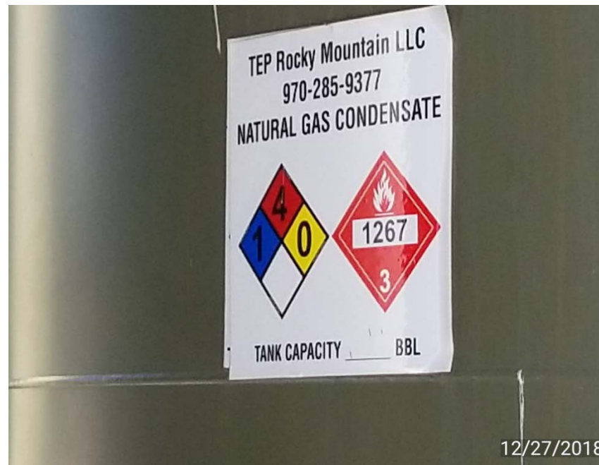
Photo 2. Tank capacity not readable.
