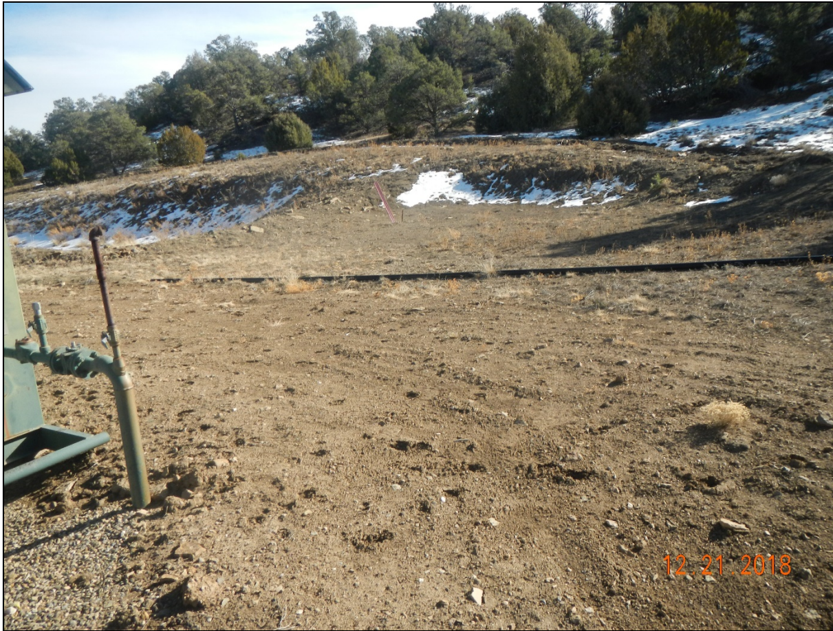
Photo 3. Facing southeast toward the cut slope. There is sparse vegetation and the soils are susceptible to erosion.
