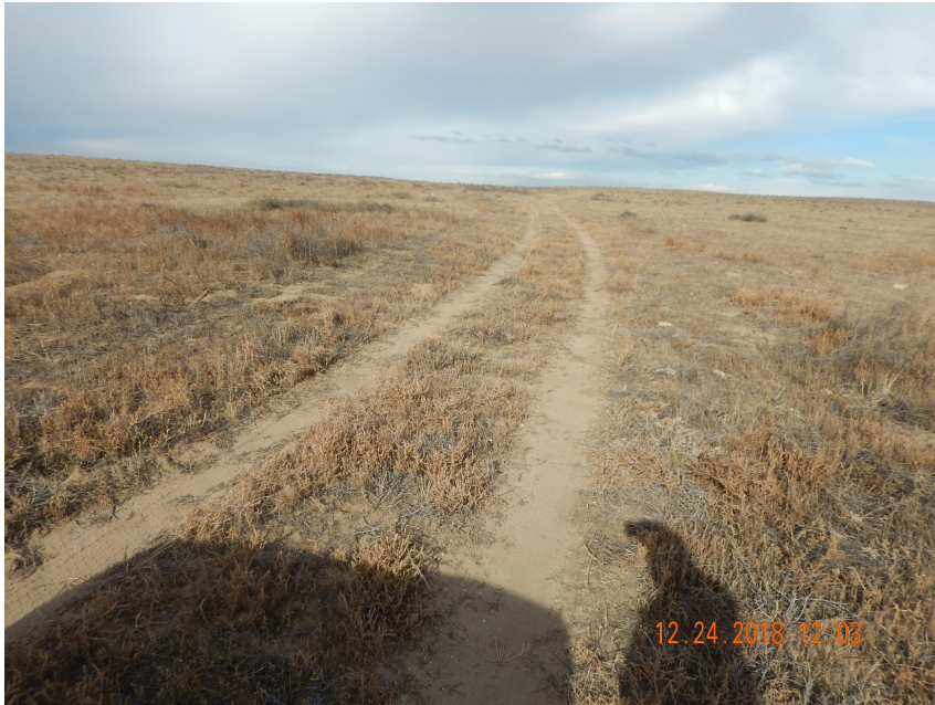
Photo 1. Photo taken from the main access road (shown in the aerial image), facing North. Operator has failed to reclaim the access road per Rule 1004 standards (e.g., recontour, decompact, etc.). Wind erosion and Russian thistle, annual weed, was observed along portions of the main access road.
