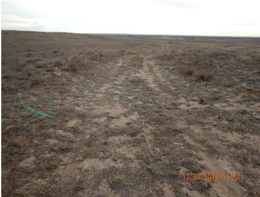
Photo 2. Photo taken from the northern well location access road, facing South. Operator has failed to reclaim the well location access road per Rule 1004 standards (e.g., recontour). Patches of Russian thistle were observed along portions of the access road and bare patches with no vegetation.
