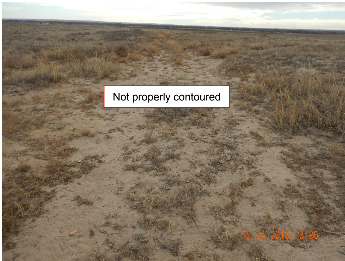
Photo 3. Photo taken from the northern well location access road, facing South. Operator has failed to reclaim the well location access road per Rule 1004 standards (e.g., recontour). Patches of Russian thistle were observed along portions of the access road and bare patches with no vegetation.
