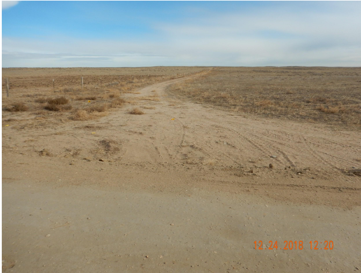
Photo 1. Photo taken from the northwestern main access road (shown in the first aerial image), facing East. Operator has failed to reclaim the access road per Rule 1004 standards (e.g., recontour, decompact, etc.). Wind erosion was observed along portions of the main access road.
