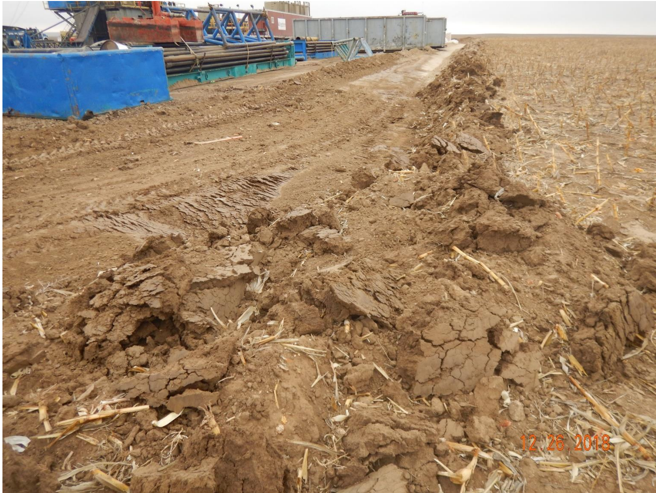
Photo 7: Photo taken from the northeast corner of the location, facing west Photo shows a sotrmwater ditch has been constructed along the perimeter of the pad. Ditch does not appear to have been constructed with good engineering practices; ditch walls have not been compacted with unconsolidated soils left as a “berm”.
