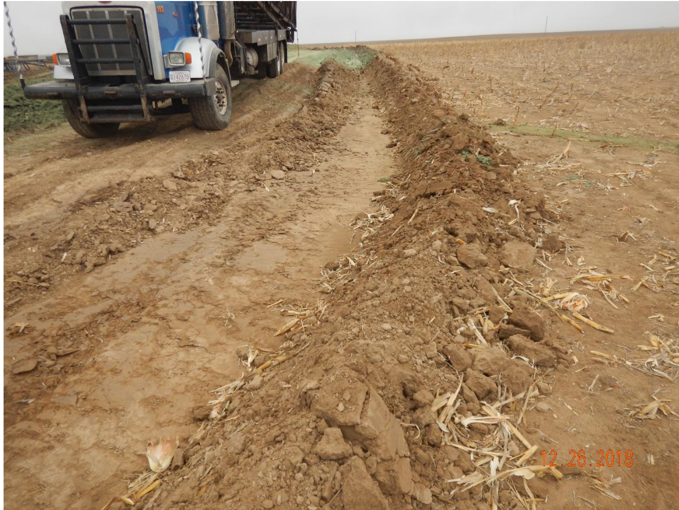
Photo 3: Photo taken from the southwest corner of the location, facing east. Photo shows a sotrmwater ditch has been constructed along the perimeter of the pad. Ditch does not appear to have been constructed with good engineering practices; ditch walls have not been compacted with unconsolidated soils left as a “berm”.
