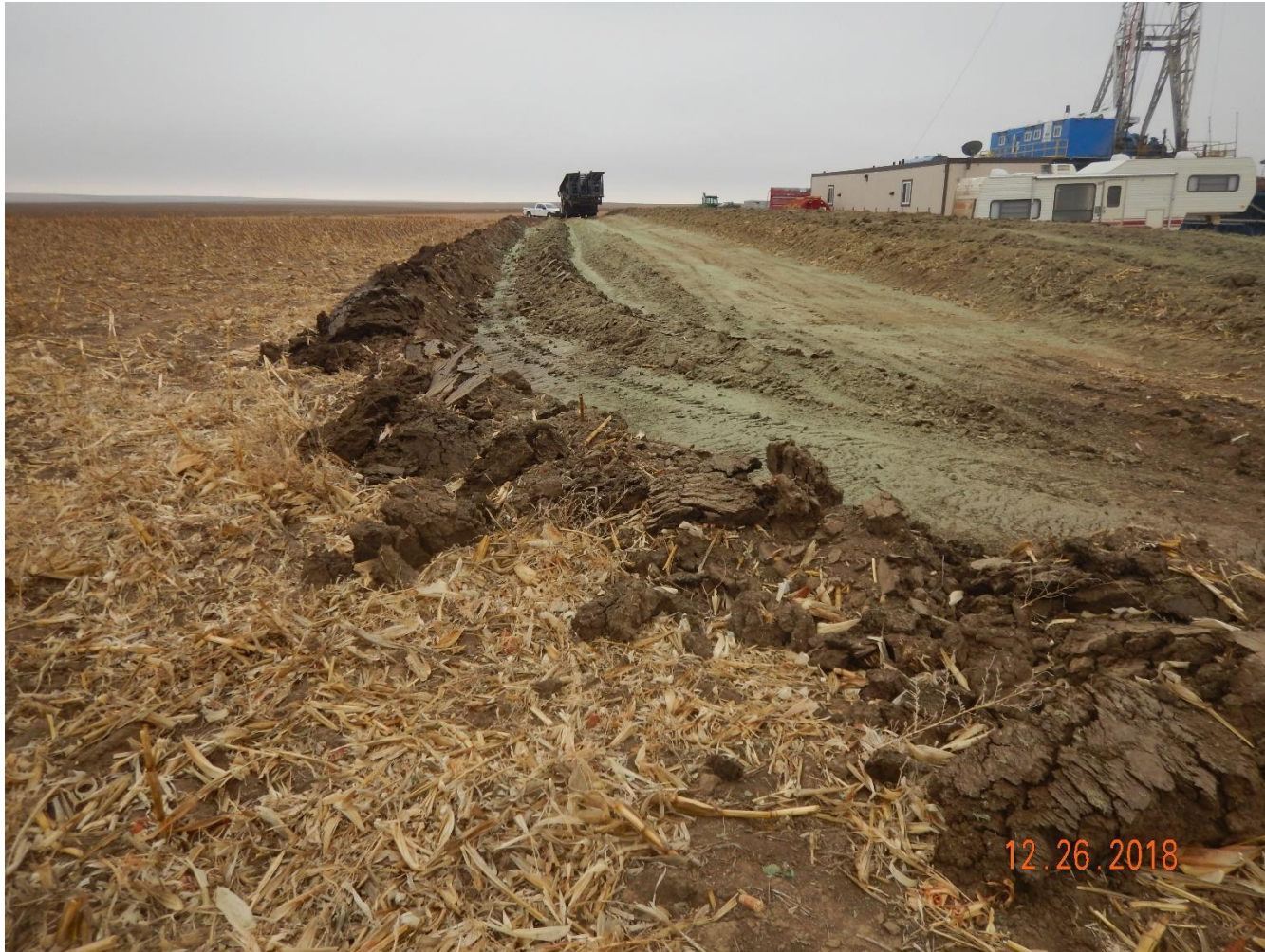
Photo 4: Photo taken from the southeast corner of the location, facing west Photo shows a sotrmwater ditch has been constructed along the perimeter of the pad. Ditch does not appear to have been constructed with good engineering practices; ditch walls have not been compacted with unconsolidated soils left as a “berm”.
