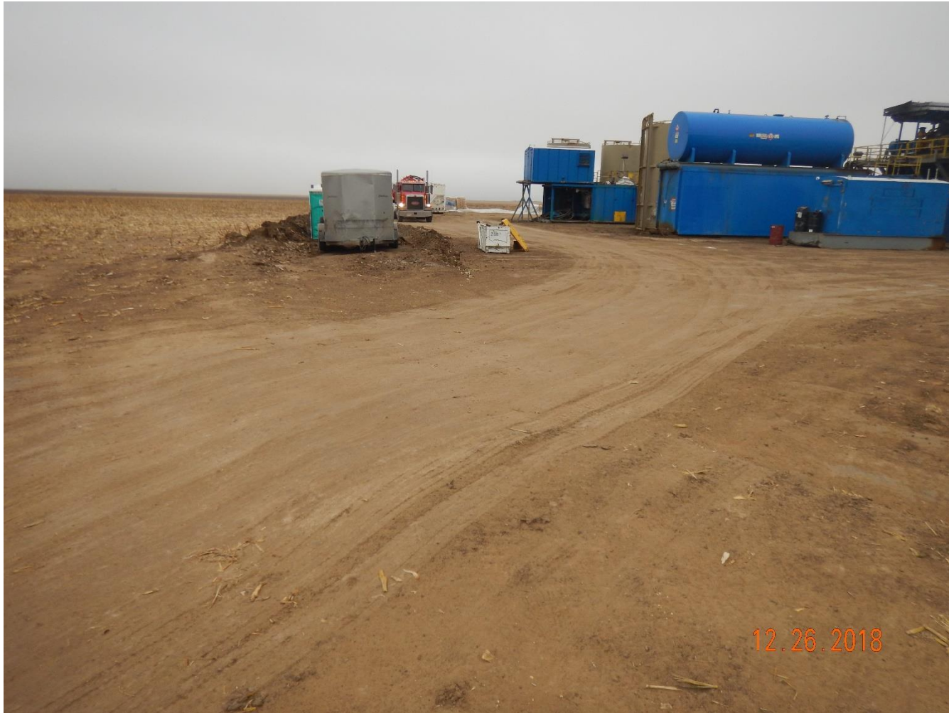
Photo 1: Photo taken from the southwest corner of the location, facing north. Photo shows a sotrmwater ditch has been constructed along the perimeter of the pad.
