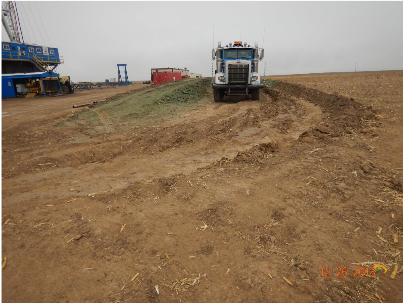
Photo 2: Photo taken from the southwest corner of the location, facing east. Photo shows a sotrmwater ditch has been constructed along the perimeter of the pad. Ditch does not appear to have been constructed with good engineering practices.
