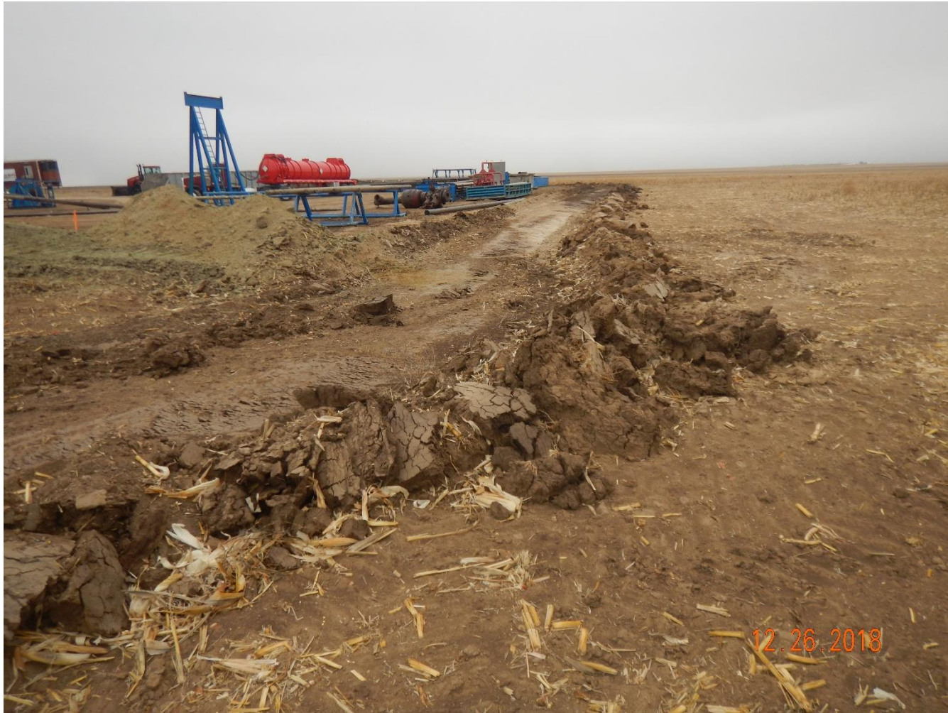
Photo 5: Photo taken from the southeast corner of the location, facing north Photo shows a sotrmwater ditch has been constructed along the perimeter of the pad. Ditch does not appear to have been constructed with good engineering practices; ditch walls have not been compacted with unconsolidated soils left as a “berm”.
