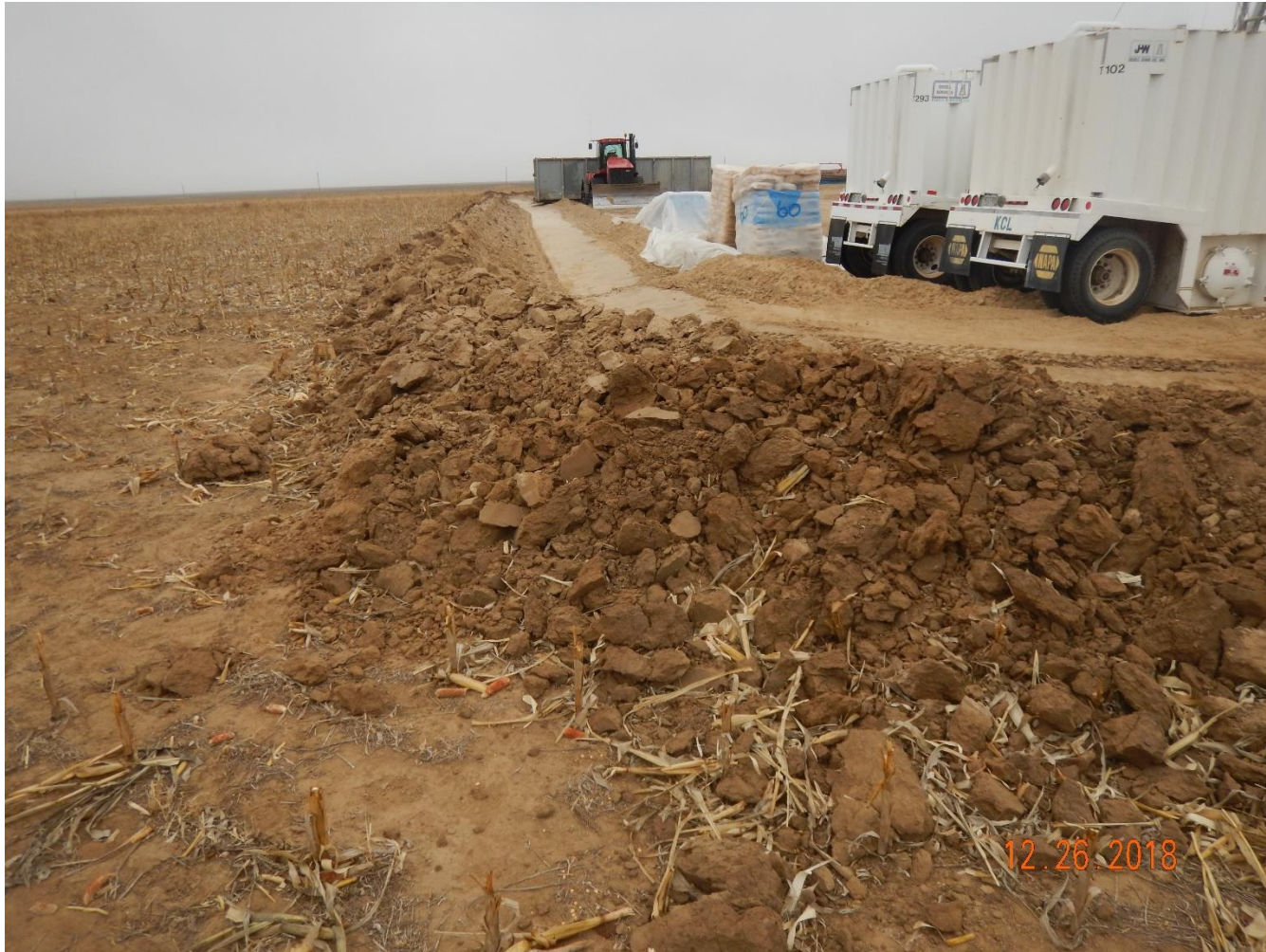
Photo 8: Photo taken from the northwest corner of the location, facing east Photo shows a sotrmwater ditch has been constructed along the perimeter of the pad. Ditch does not appear to have been constructed with good engineering practices; ditch walls have not been compacted with unconsolidated soils left as a “berm”.
