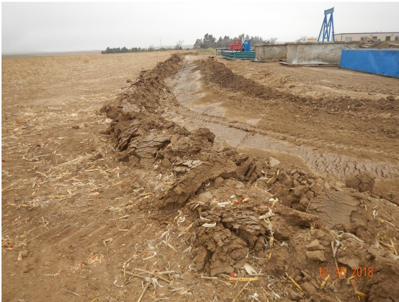
Photo 6: Photo taken from the northeast corner of the location, facing southwest. Photo shows a stormwater ditch has been constructed along the perimeter of the pad. Ditch does not appear to have been constructed with good engineering practices; ditch walls have not been compacted with unconsolidated soils left as a “berm”.
