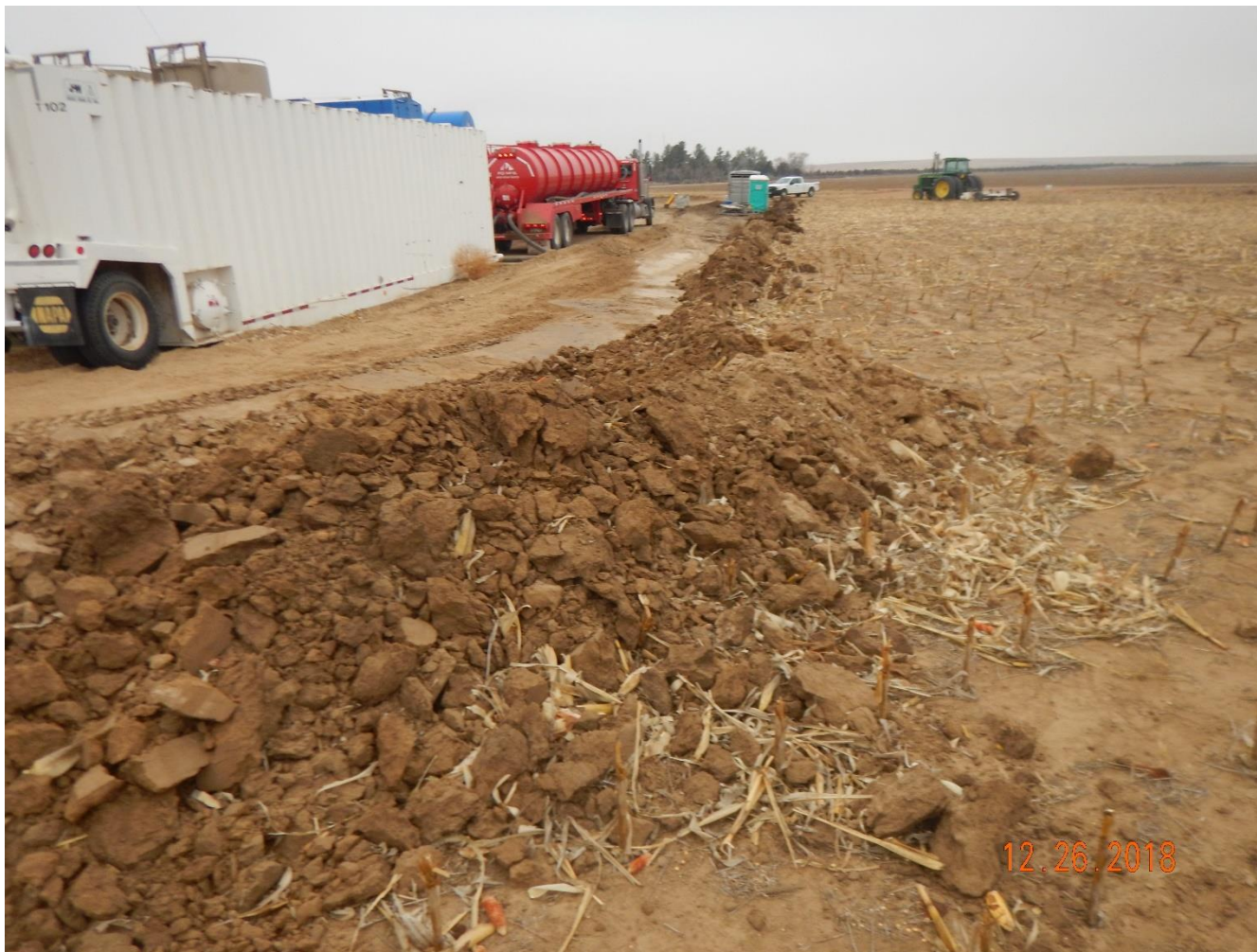
Photo 9: Photo taken from the northwest corner of the location, facing southwest. Photo shows a stormwater ditch has been constructed along the perimeter of the pad. Ditch does not appear to have been constructed with good engineering practices; ditch walls have not been compacted with unconsolidated soils left as a “berm”.
