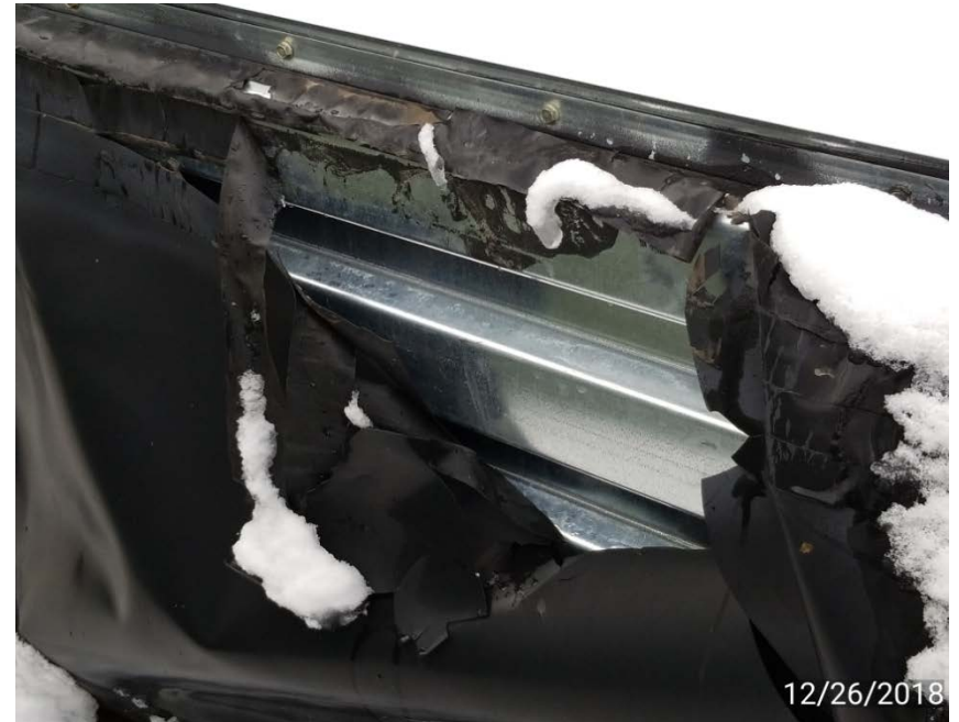
Photo 2. Tank secondary containment liner inadequate.
