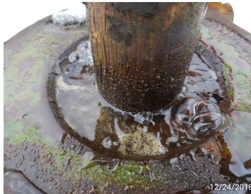
Photo 2. Well head leaking gas.
