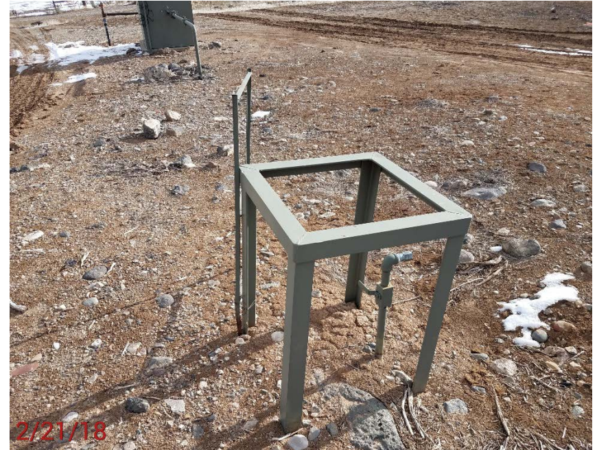
Location Photo #2, Unmarked flow line riser.
