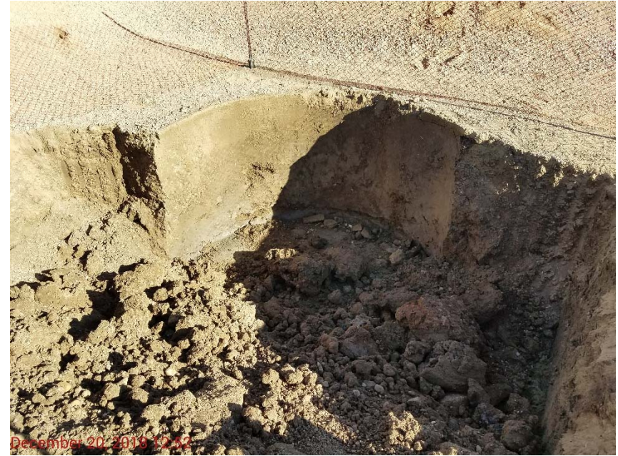
Photo 2 – Excavation/Footprint of removed produced water vessel.
