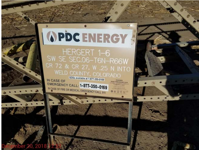
Photo 1 – Hergert 1-6 Tank Battery
