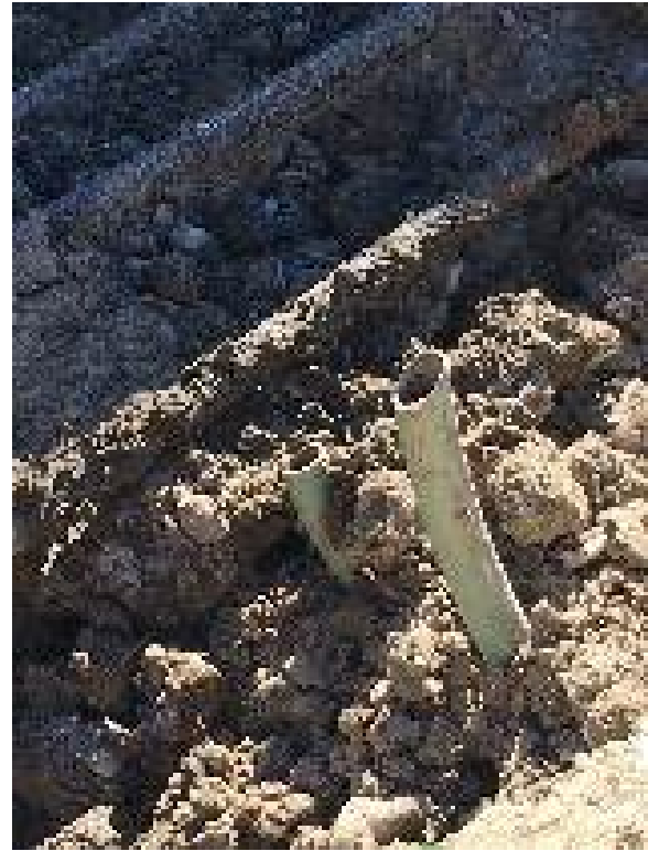
Flowlines in exaction trench with 2 other Abandoned flowlines discovered when digging. They were open ended
