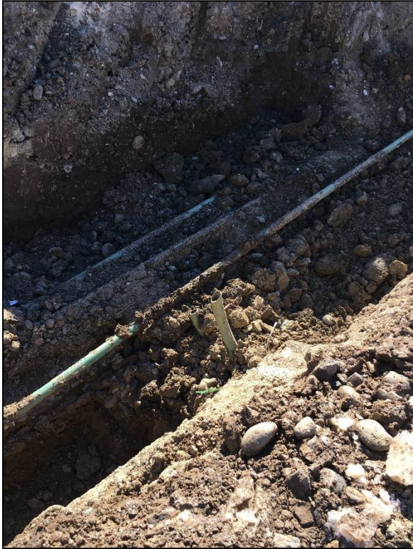
Flowlines in exaction trench with 2 other Abandoned flowlines discovered when digging. They were open ended
