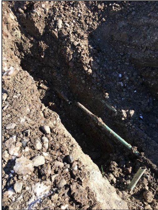
Flowlines pictured in excavation
