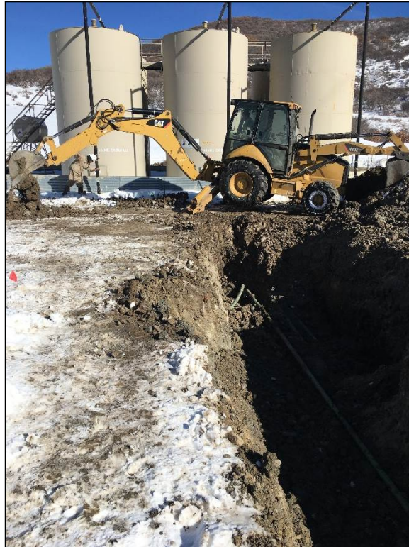
Spill area, Flowline with leak travels to the tanks on right side
