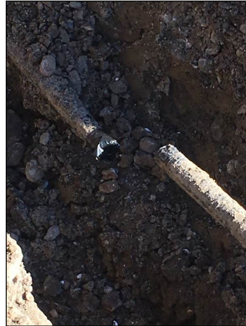
Flowline with section cut out where leak was found
