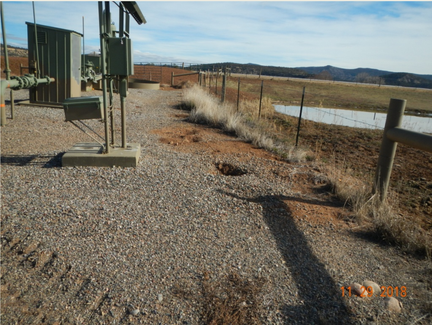
Photo 3. View of the southern project area from the southeastern corner facing westward.
