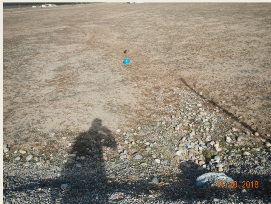
Photo 6. View of area downstream of culvert, erosional downcutting up to 1.5 feet deep and 3 feet wide observed. Stabilization is needed.
