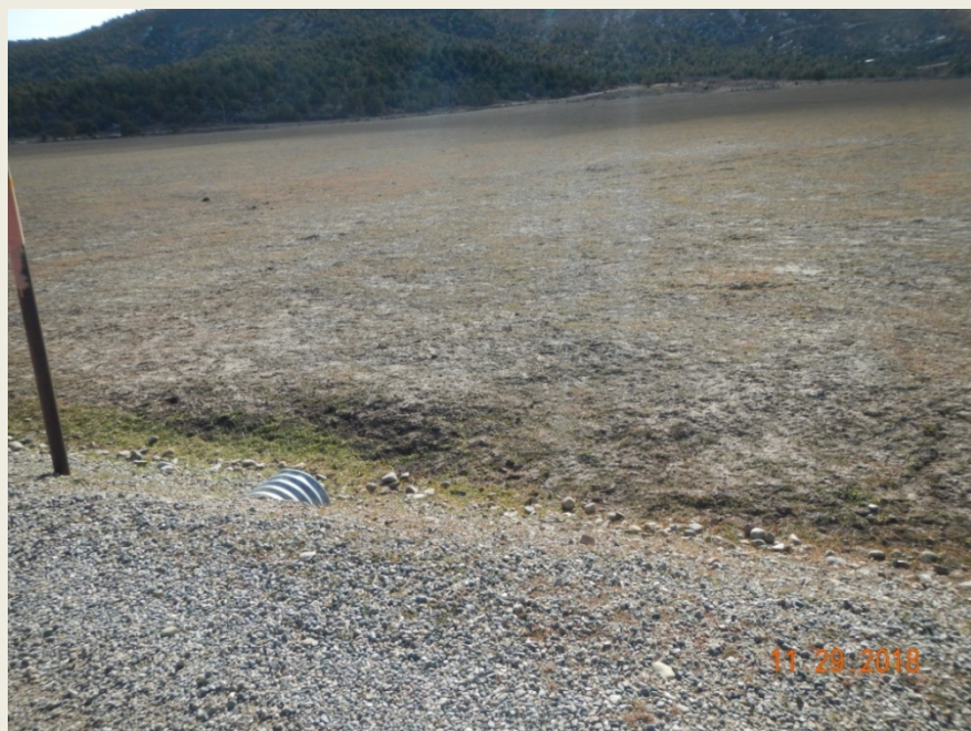
Photo 5. View of area upstream of culvert, no down-cutting observed.
