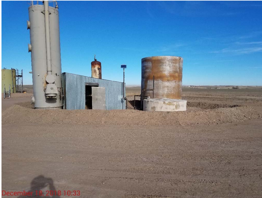
Photo 3 – Heater Treat and produced water tanks, Hoffman 34-10
