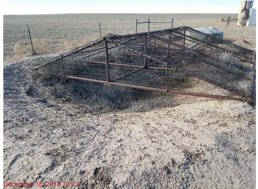
Photo 4 – East side of Macaw 33-1 produced water pit showing gap in netting coverage.
