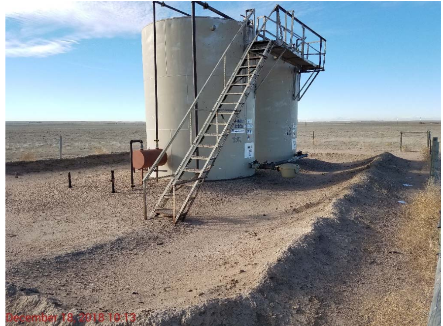
Photo 2 – Federal Falcon 33-6 tank battery, secondary containment requires maintenance
