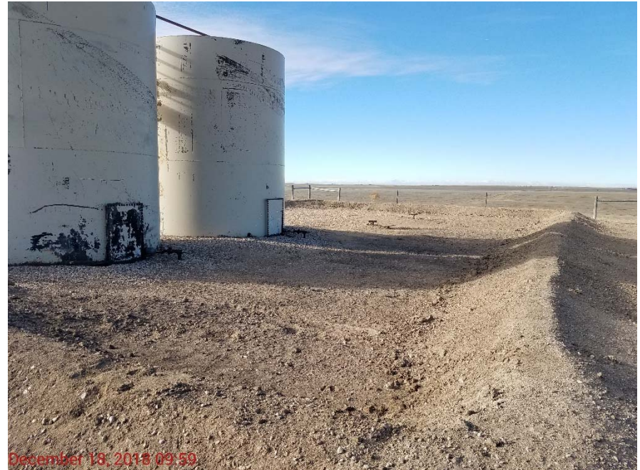
Photo 2 – Rear and repaired containment at Federal Goshawk 28-13 tank battery
